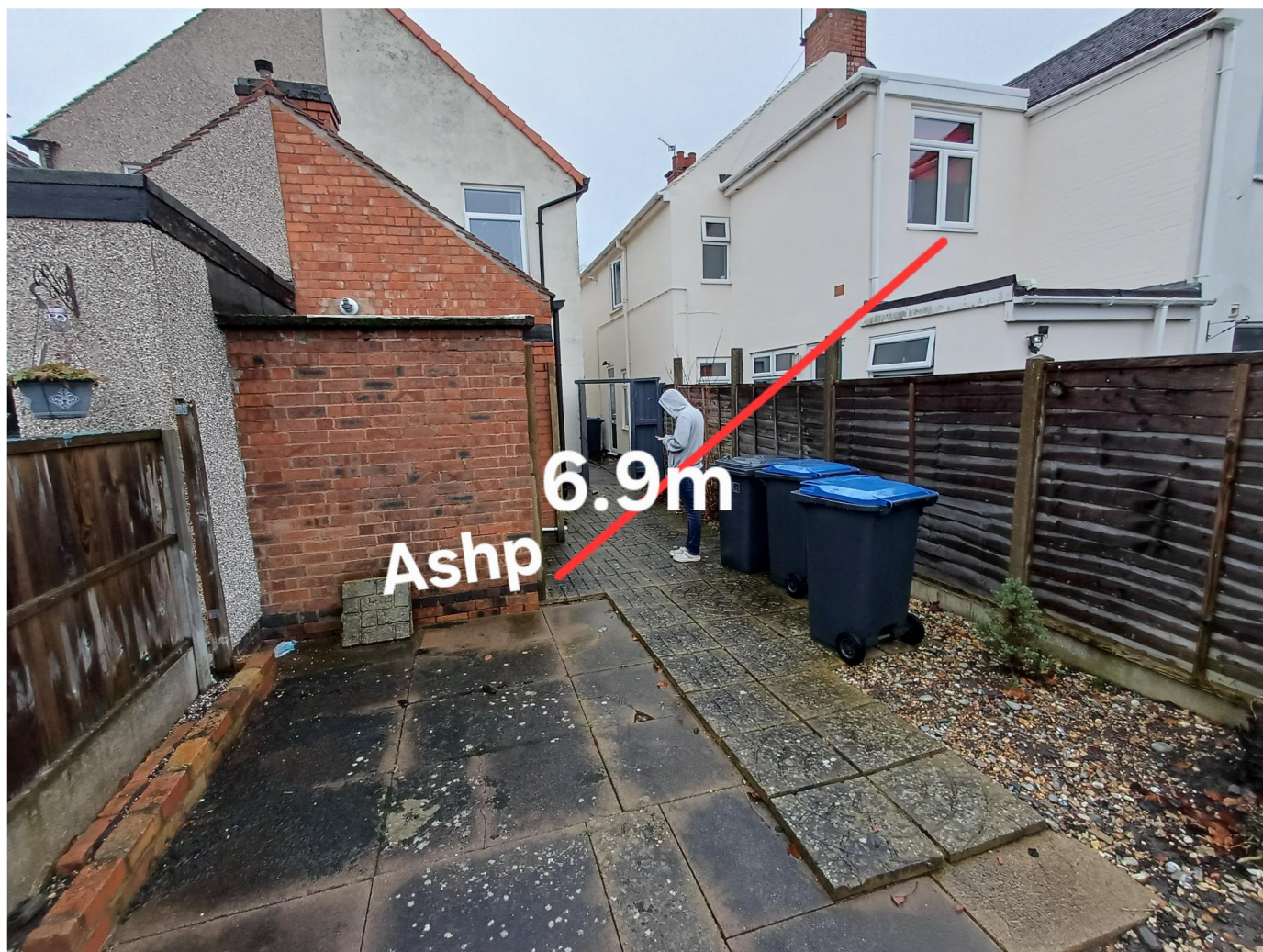
Annotated Planning Application Photo
