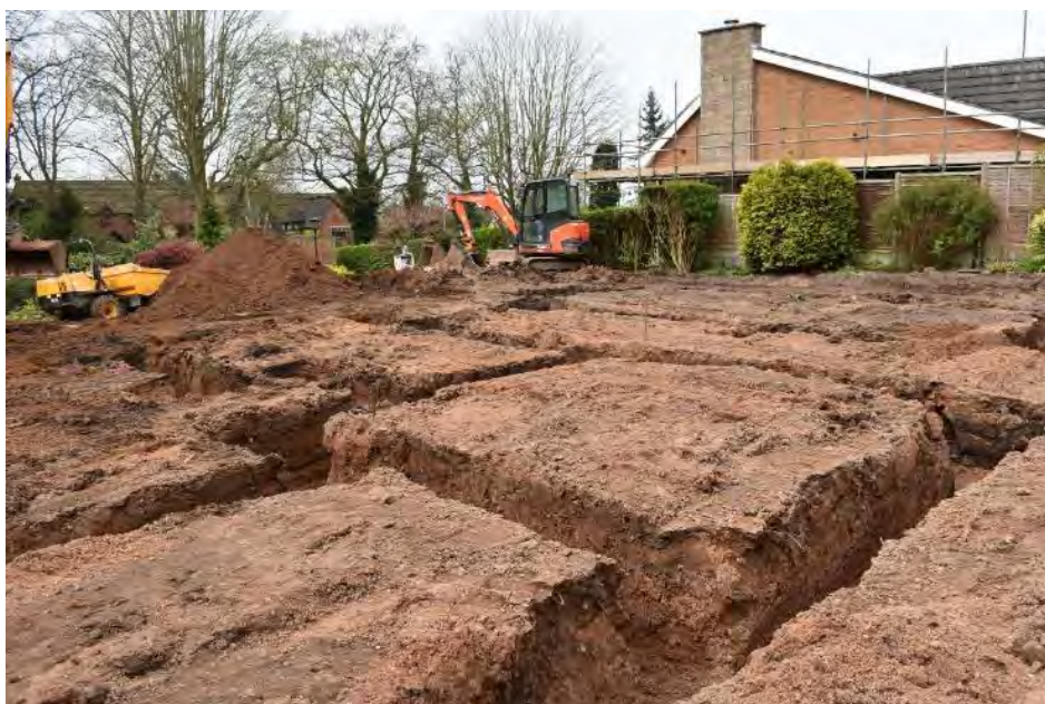
3 Excavated foundation trenches looking north-west
