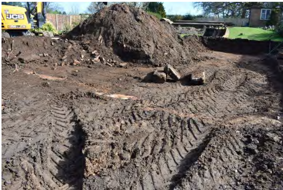
2 Working shot of ground reduction looking north-east
