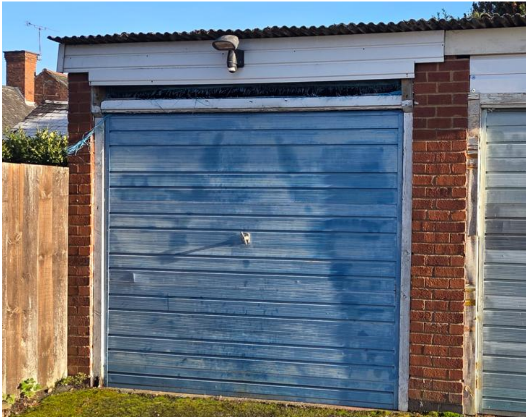
Photograph 6: Gap above the garage door.
