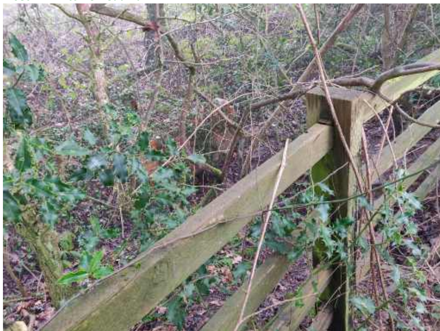
Inset 2.1: Ditch C Headwall
