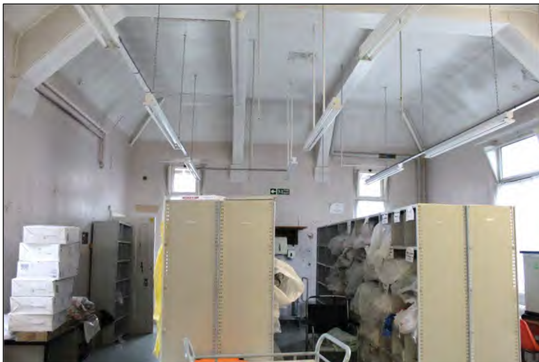
Photo 102 View of G60, the former Pritchard ward room, before the asbestos strip
