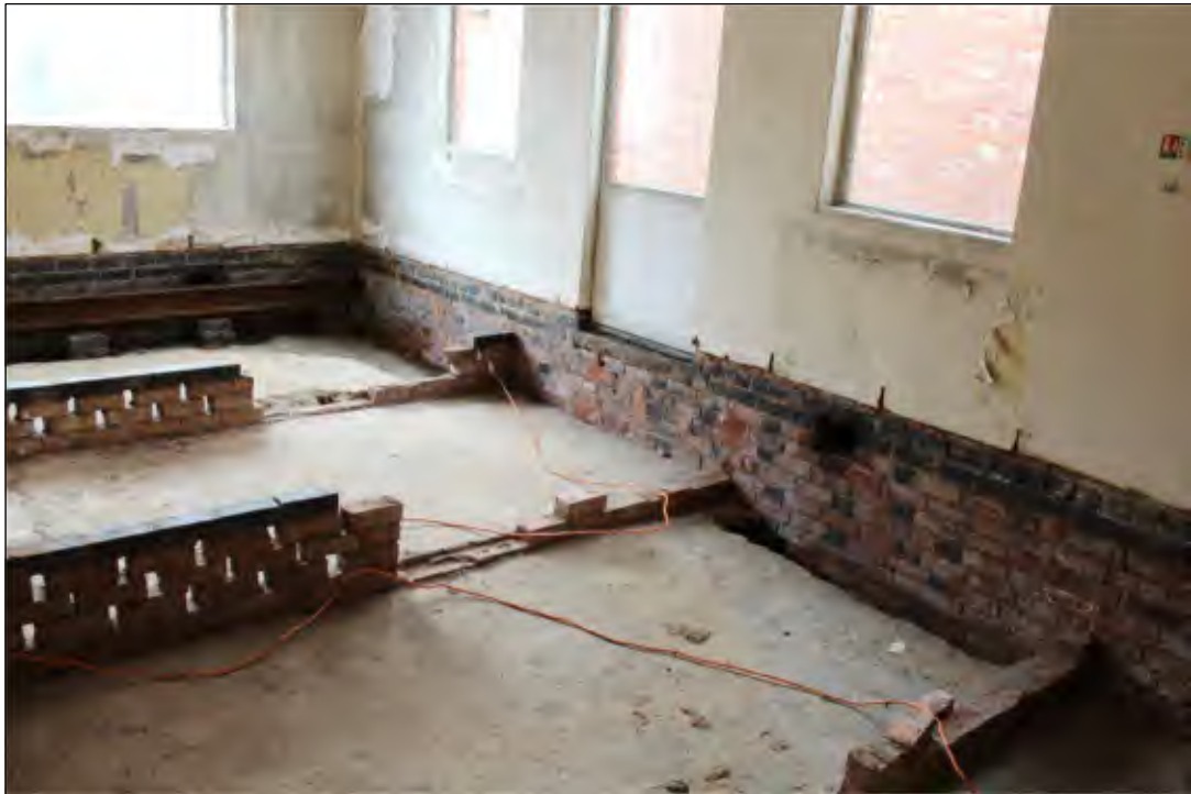
Photo 50 View of G4, former dining room, showing floor detail after asbestos strip
