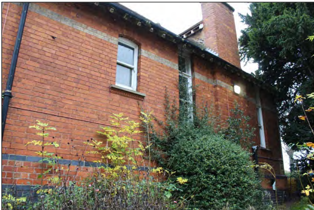
Photo 21 South-west elevation: 1900 phase, exterior of ward
