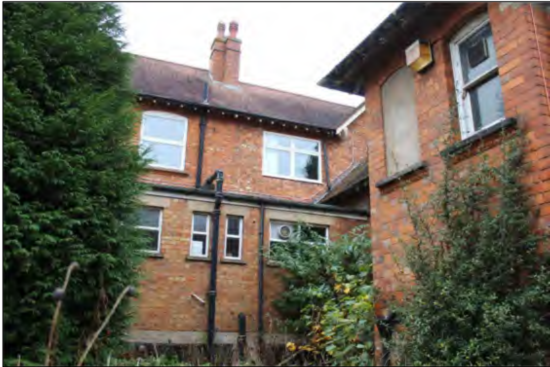
Photo 20 South-west elevation: 1900 phase, looking south-east
