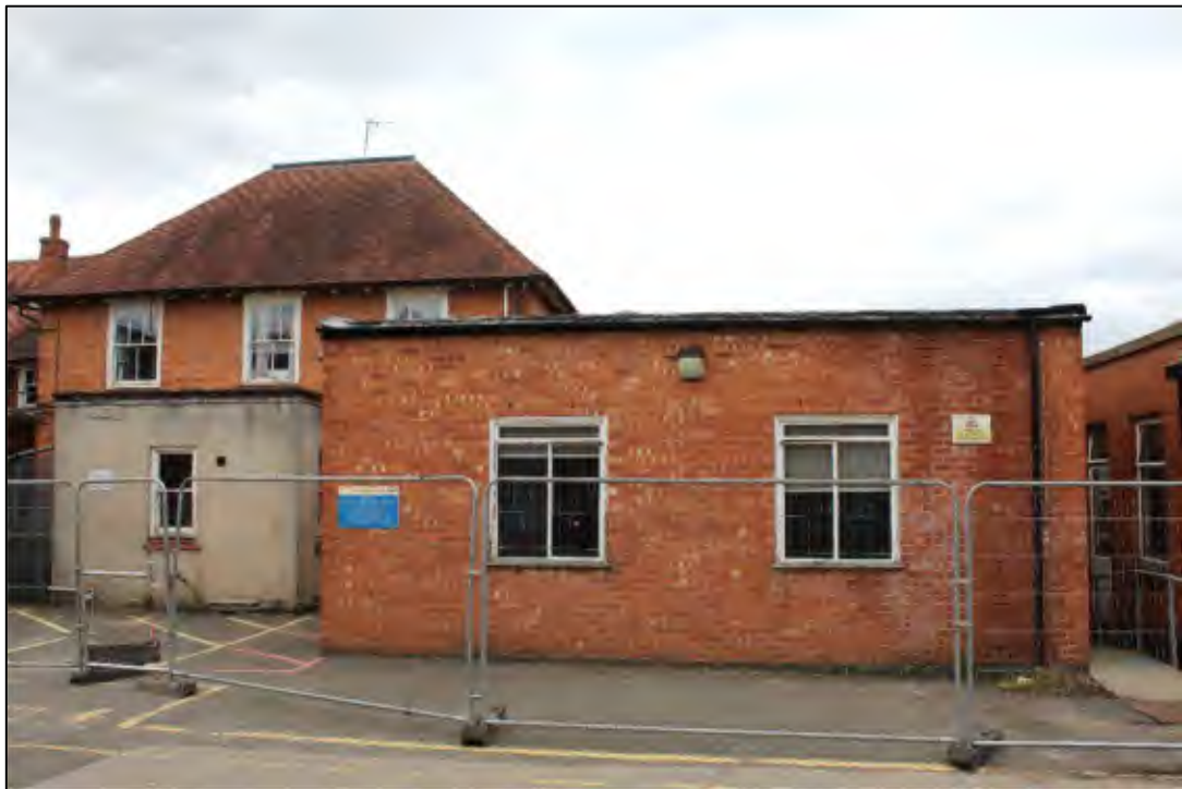
Photo 27 North-east elevation: 1938 phase, central section formed of the x-ray department
