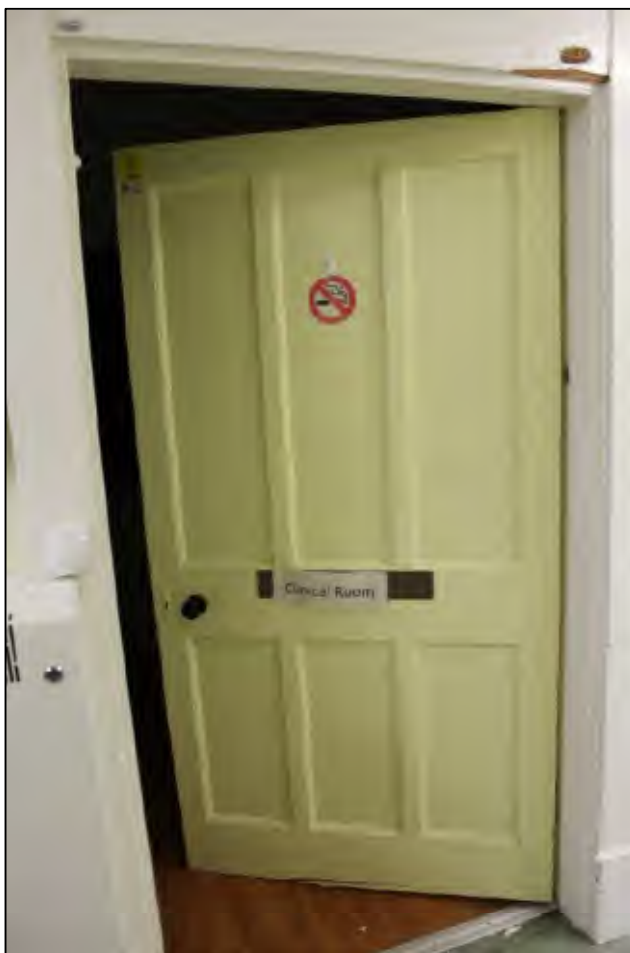
Photo 89 Entrance to room G53
