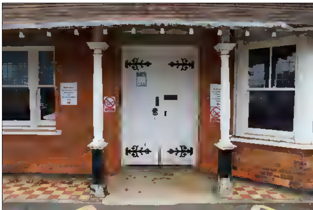
Photo 7 Principal (south-east) elevation: entrance doors
