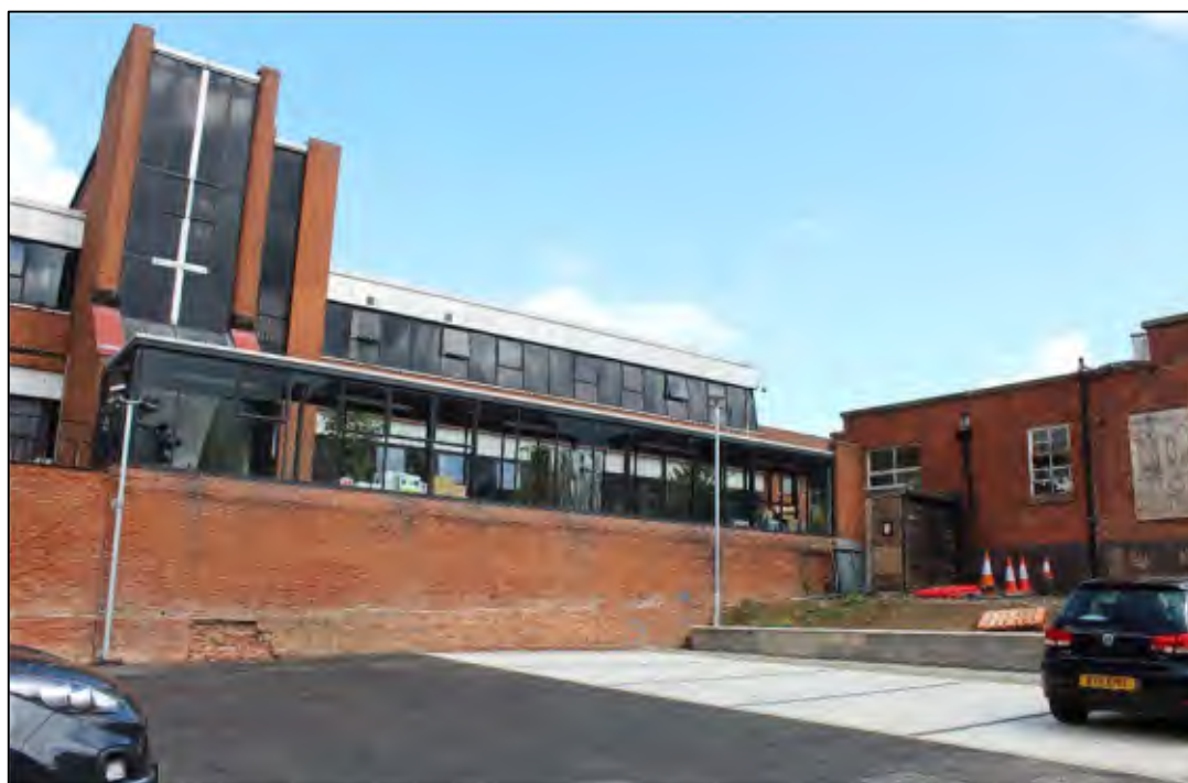
Photo 11 South-west elevation: view of glaze link, looking north
