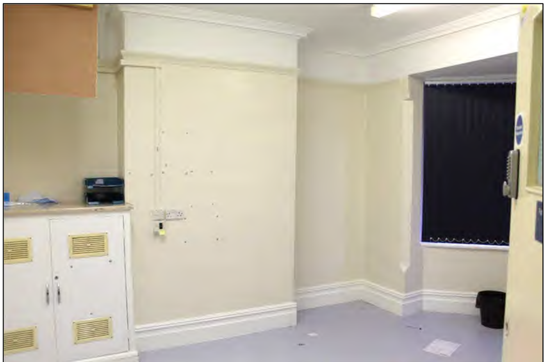
Photo 101 View of room G58, the former day room
