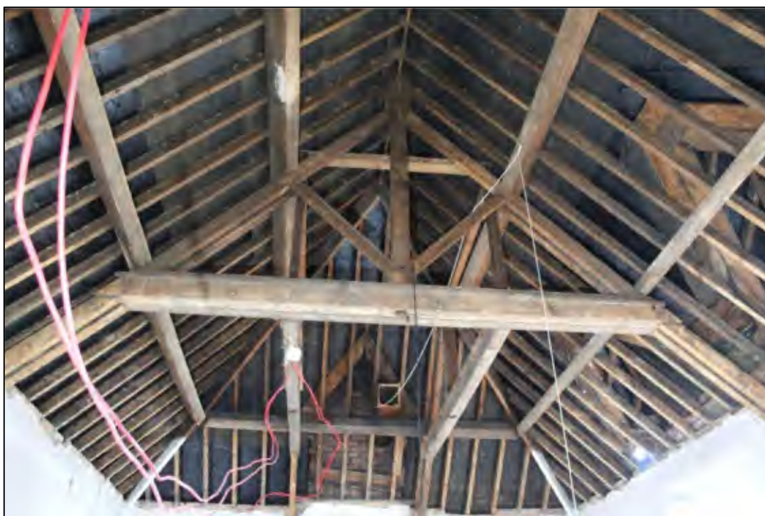
Photo 105 Detail of roof structure in room G60
