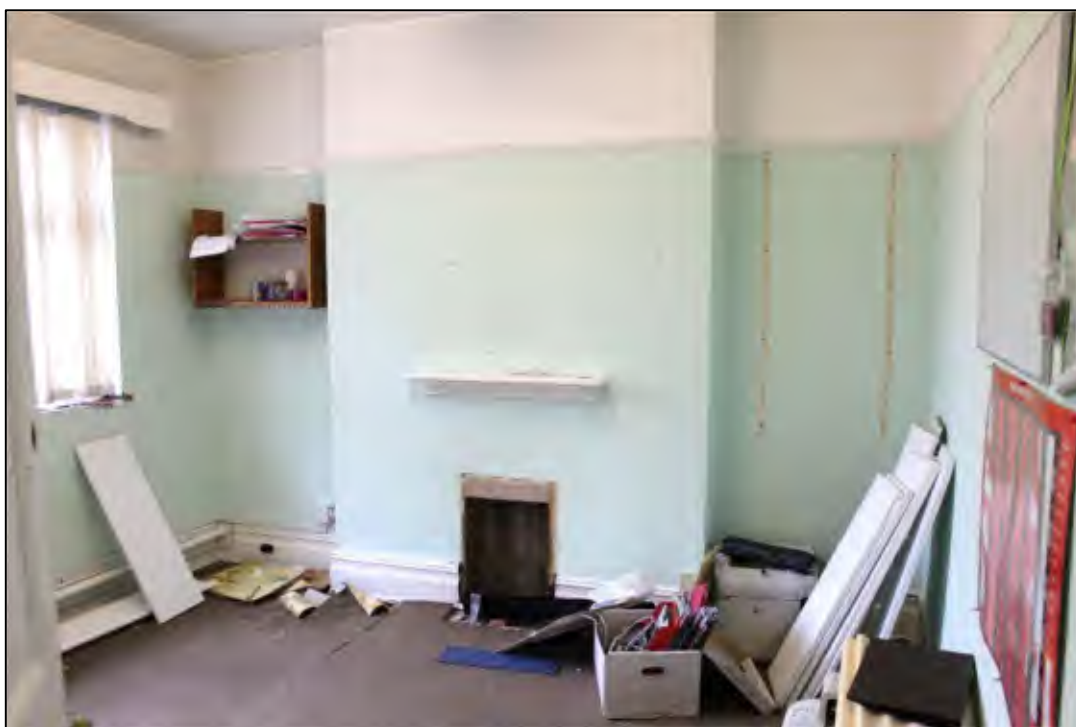
Photo 128 Overview of room F17, with fireplace removed
