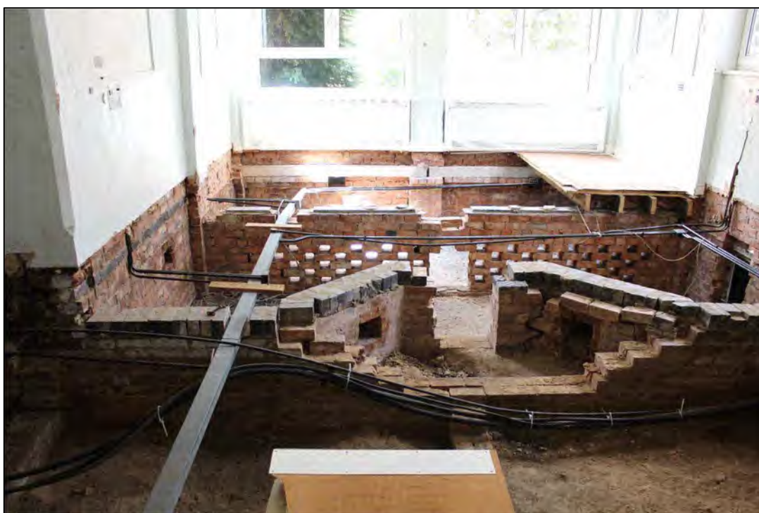
Photo 87 Detail of sub-floor structure in room G50
