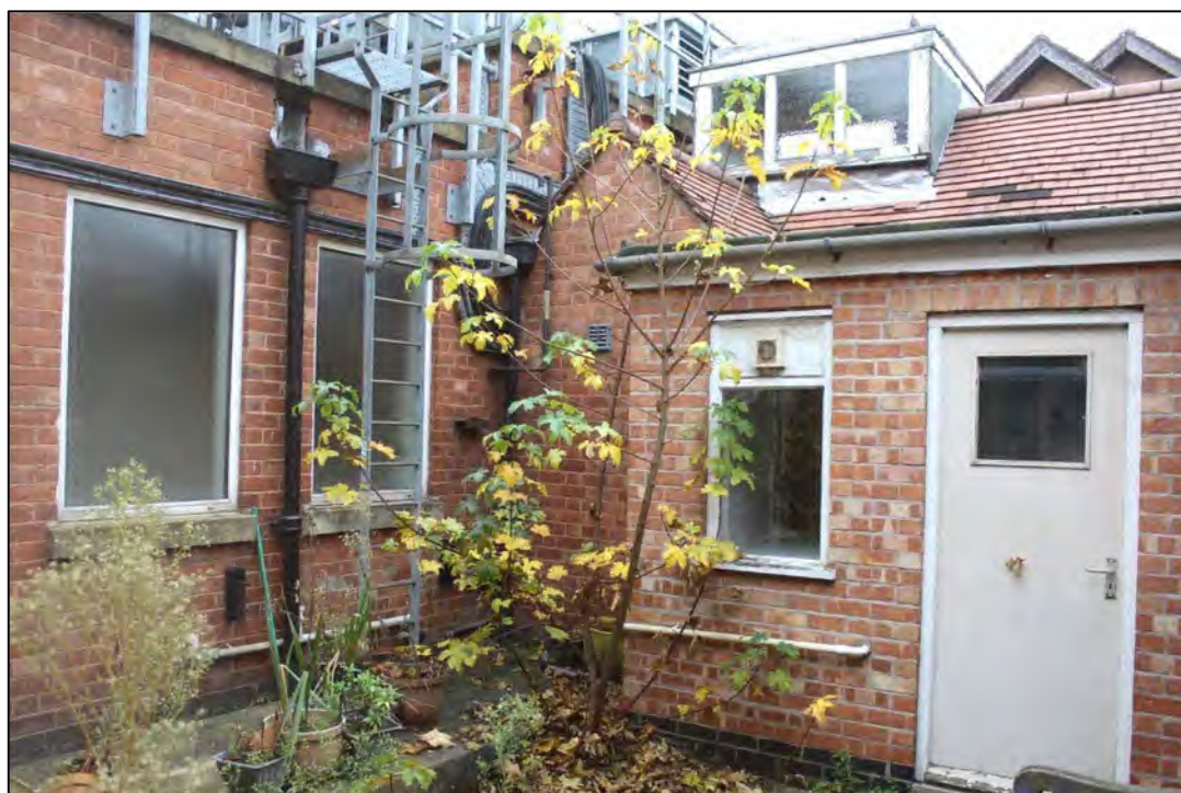
Photo 84 View of enclosed external courtyard area
