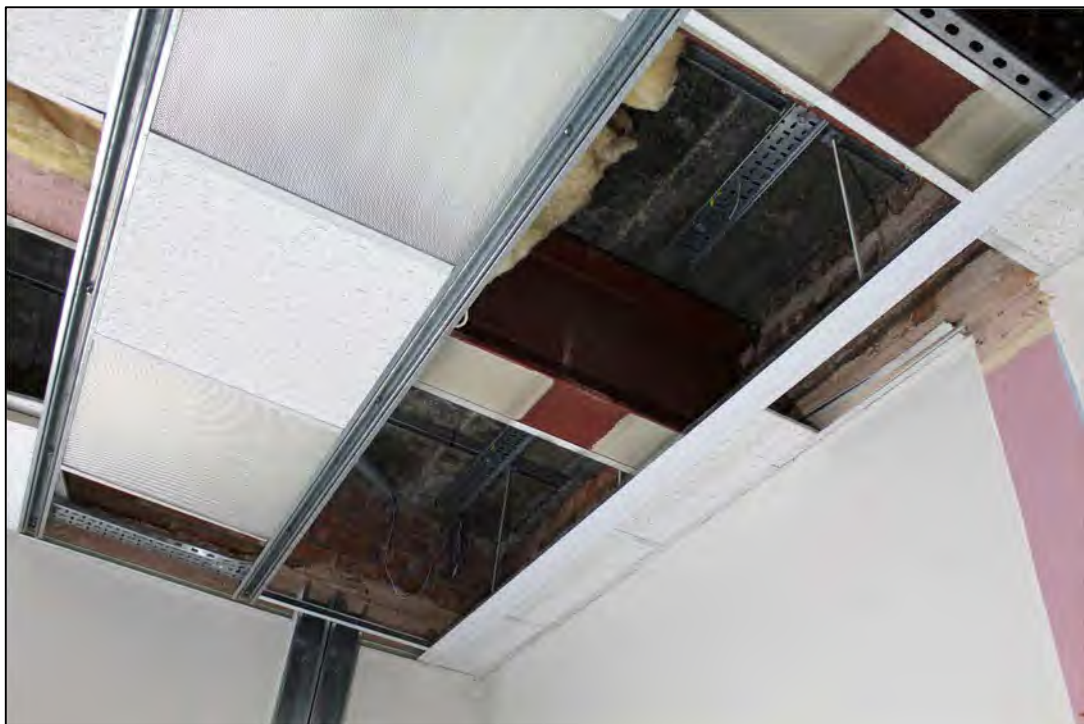
Photo 57 Detail of ceiling in G14
