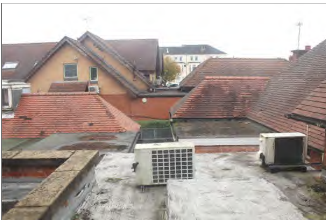
Photo 37 View of roof area on 1900 phase at first floor level (east side)
