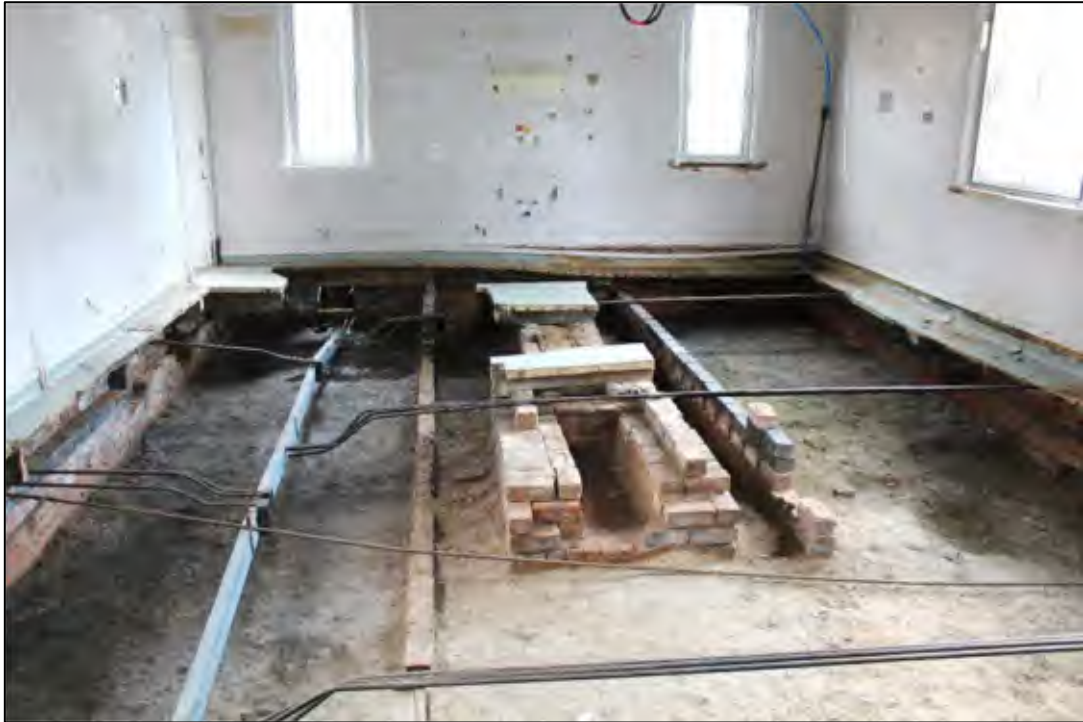
Photo 104 Detail of sub-floor structure in room G60
