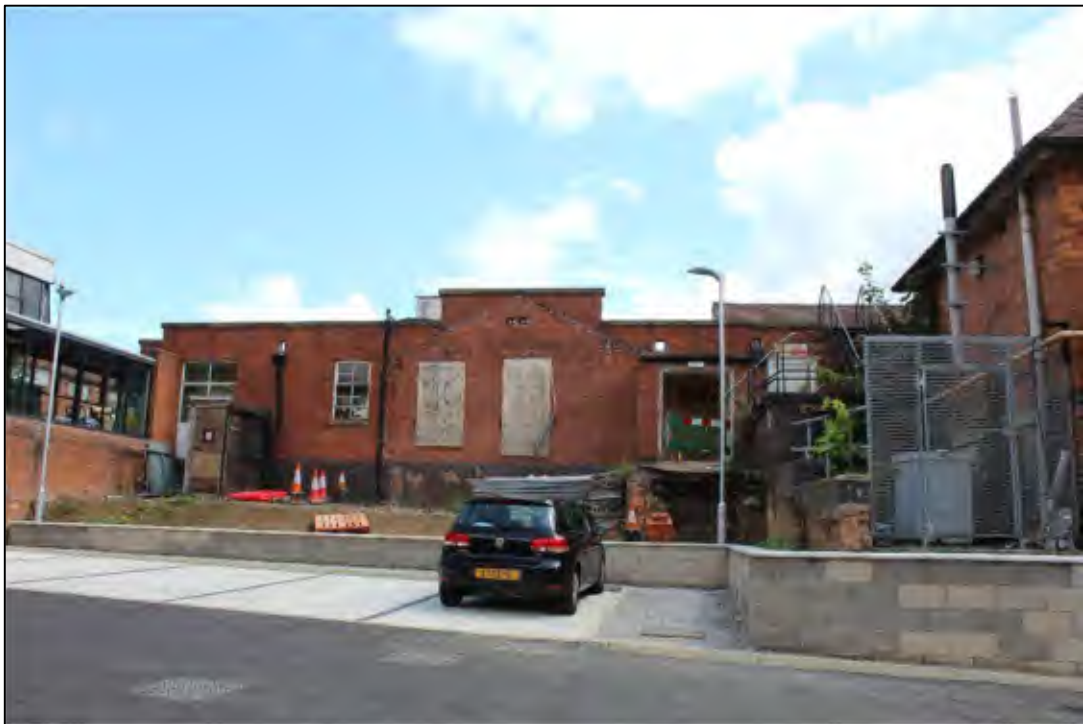
Photo 12 South-west elevation: north section (1938 phase)
