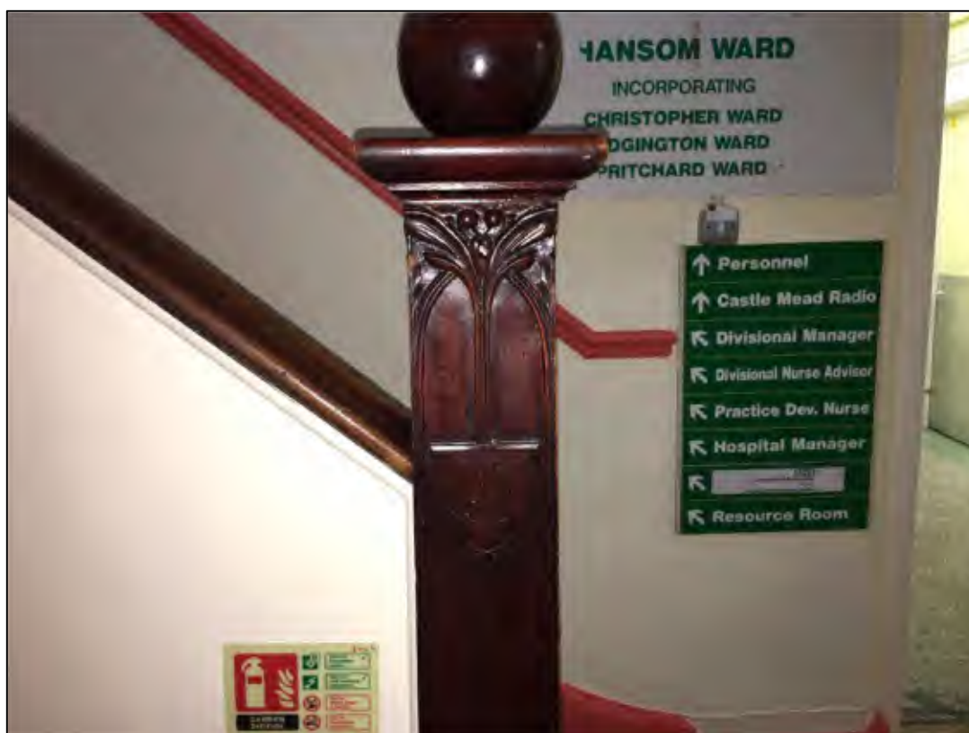
Photo 95 Detail of newel post on original 1900 staircase, looking north, with '1900' date
