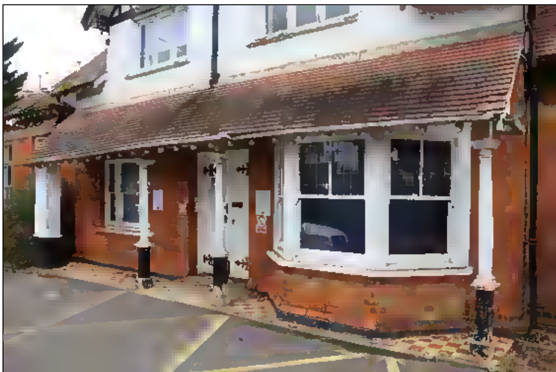
Photo 6 Principal (south-east) elevation: central entrance
