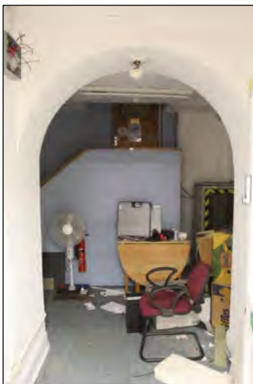
Photo 119 View of room F9, the former entrance to the Castle Mead Radio station room
