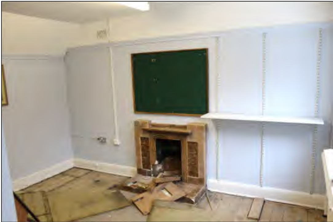
Photo 123 Overview of room F13, with timber flooring and 1930's fireplace
