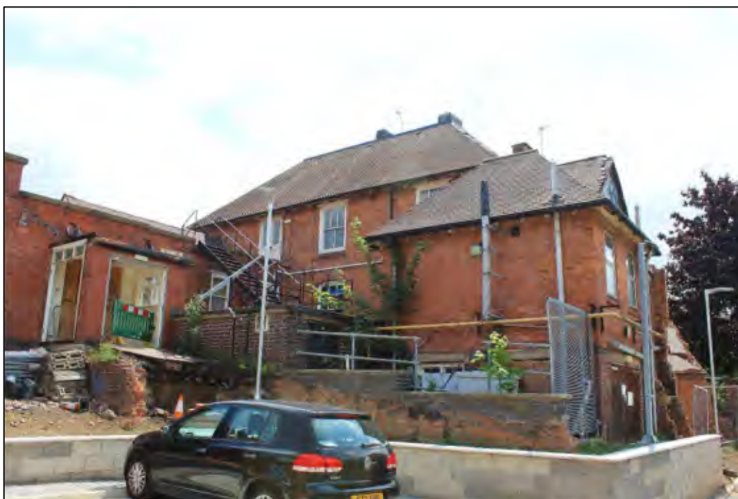
Photo 14 South-west elevation: 1938 Phase, looking south-east
