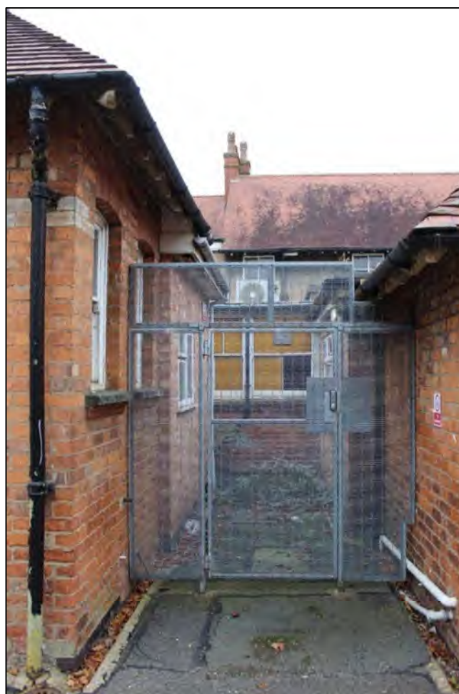
Photo 32 North-east elevation: 1900 phase, central section
