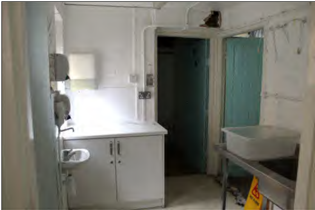
Photo 81 View of room G48, which is a post-1950's addition
