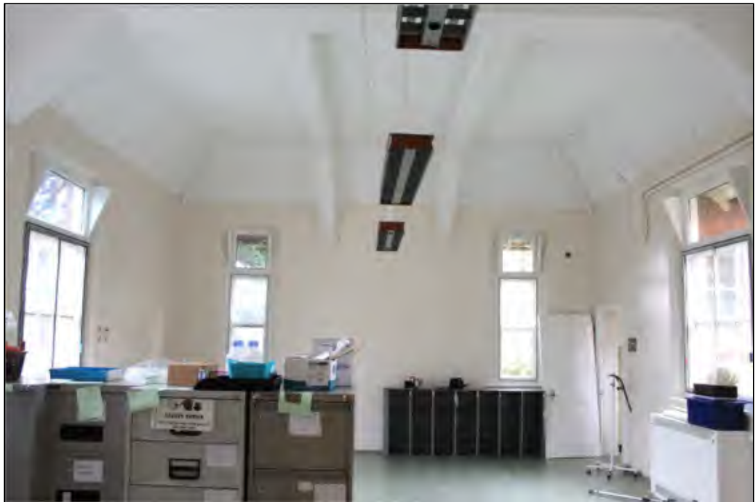
Photo 106 View of G63, the former Edington ward room, before the asbestos strip
