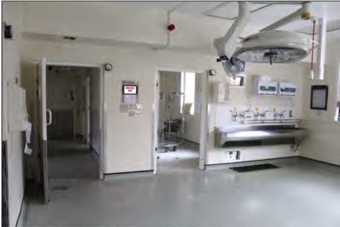
Photo 73 View of G40, the former operating theatre
