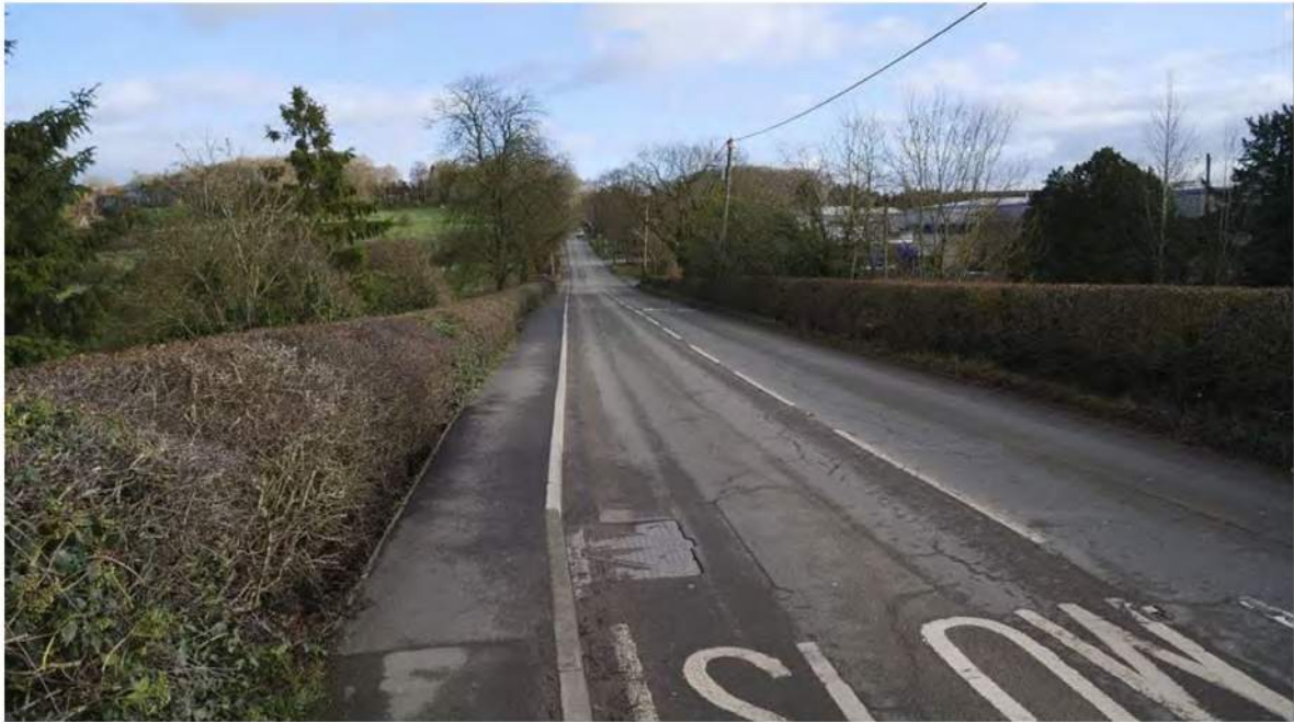
Figure 6: View 1 [Station Road Approach to Market Bosworth]
