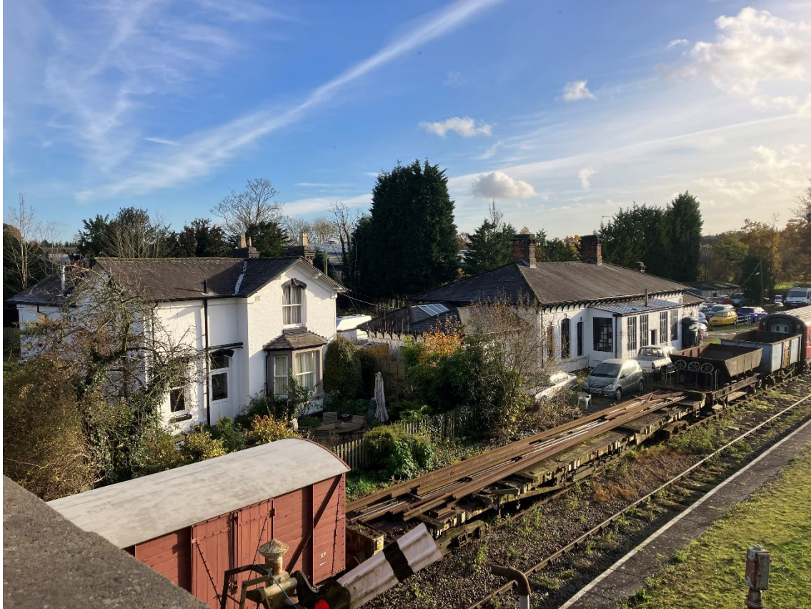
Plate 7: Looking to the south of Station Road overbridge at Station Master's House and Station of former Ashby and Nuneaton Joint Railway
