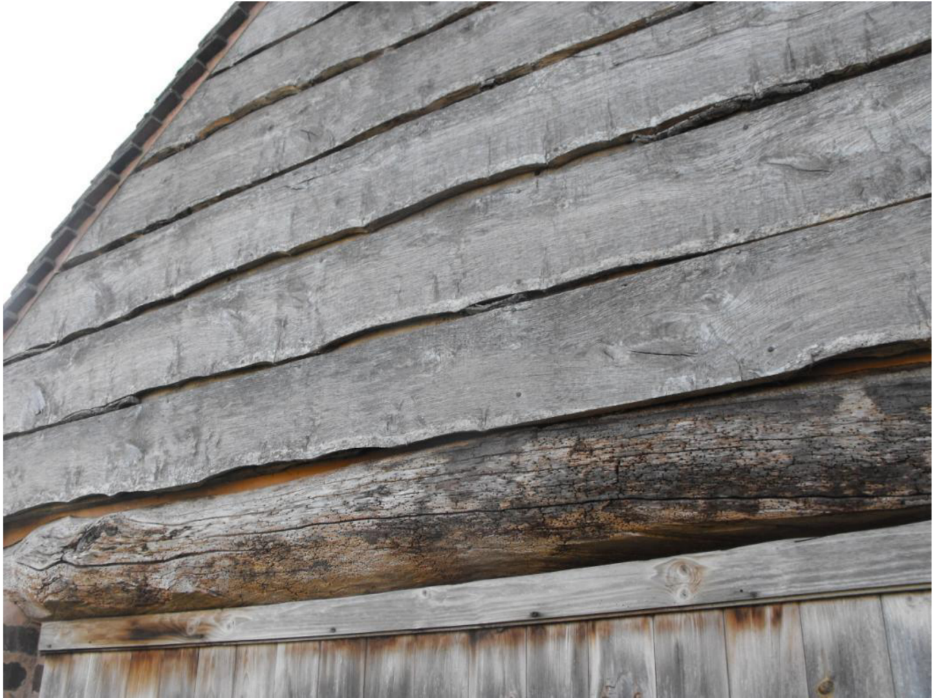
Tight fitting boarding external gables
