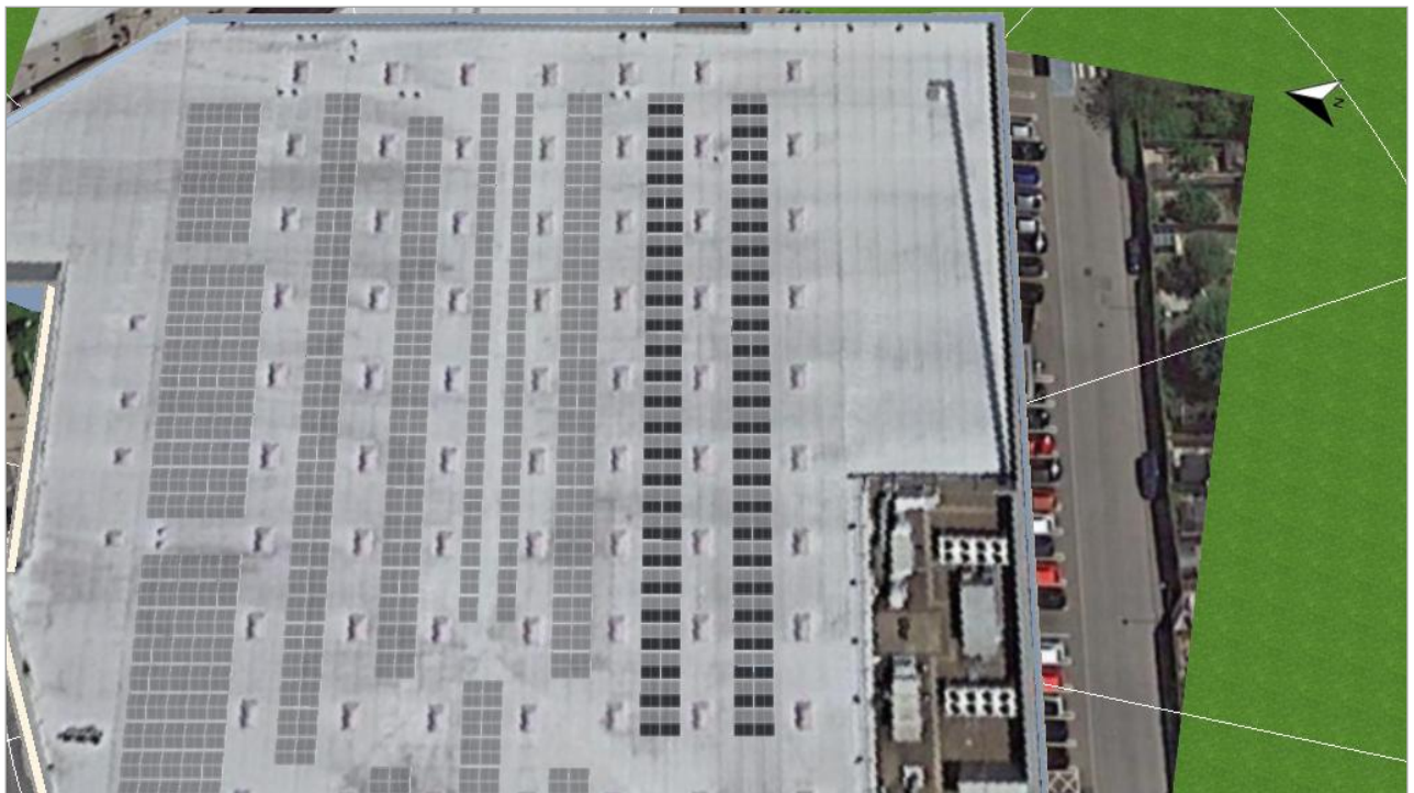
Figure: 8. Module Area - Arbitrary Building 01-Module Area West
