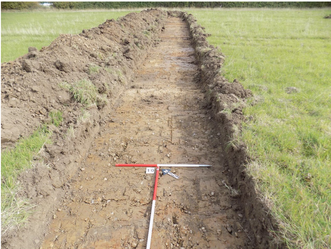
Trench 10 general shot
