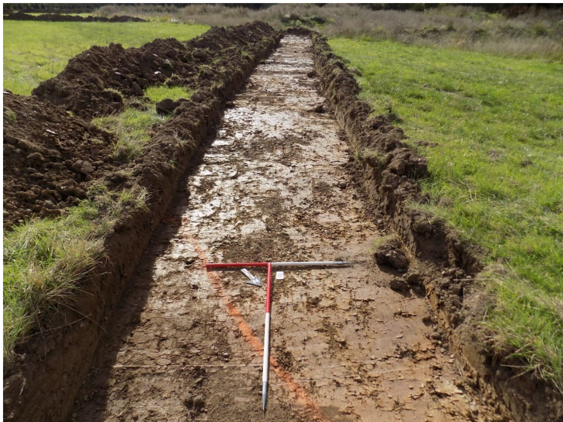
Trench 08 general shot
