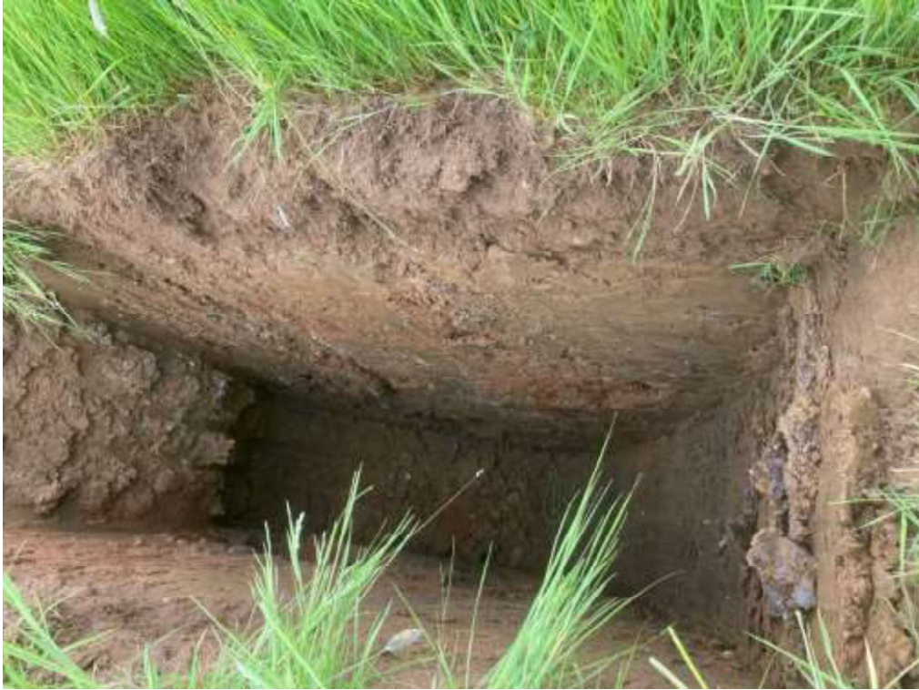
TP27 – Trial Pit
