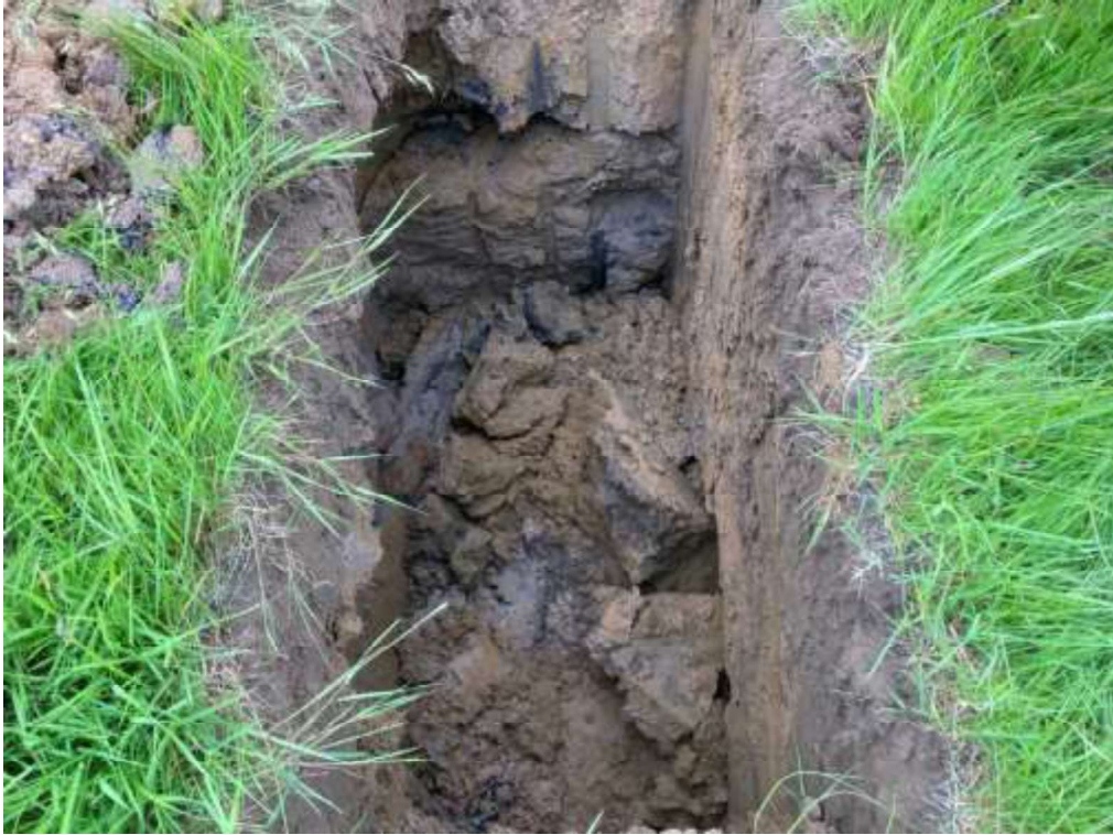
TP49 – Trial Pit
