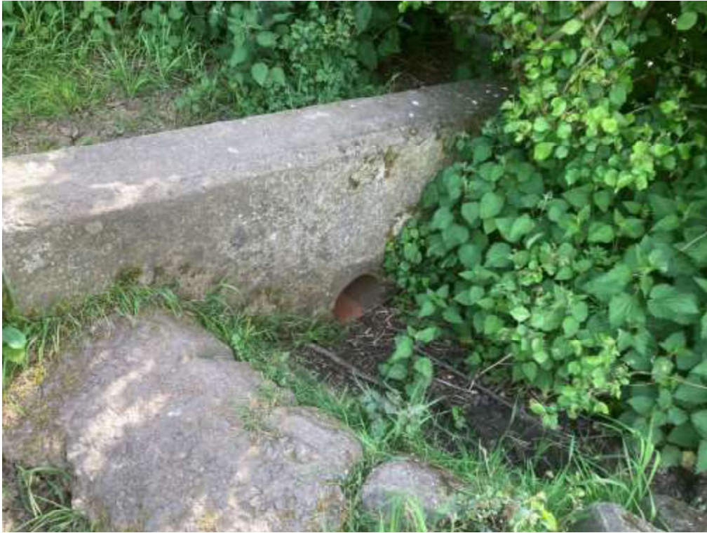
Looking south at a concrete drainage structure passing beneath the M69
