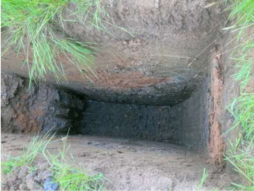
TP44 – Trial Pit
