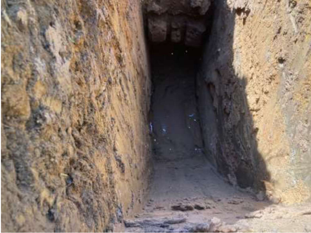
TP28 – Trial Pit
