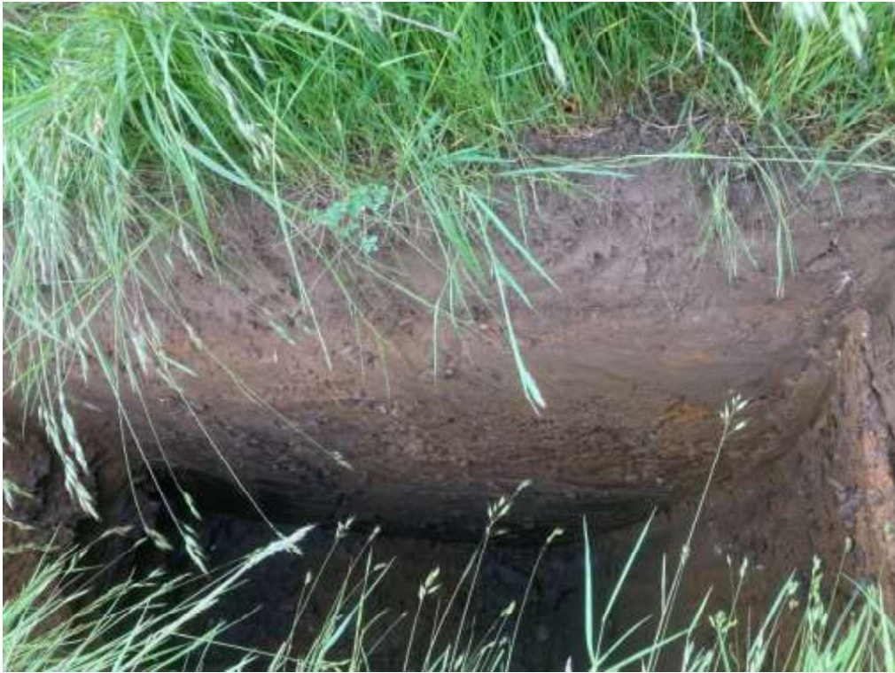
TP42 – Trial Pit
