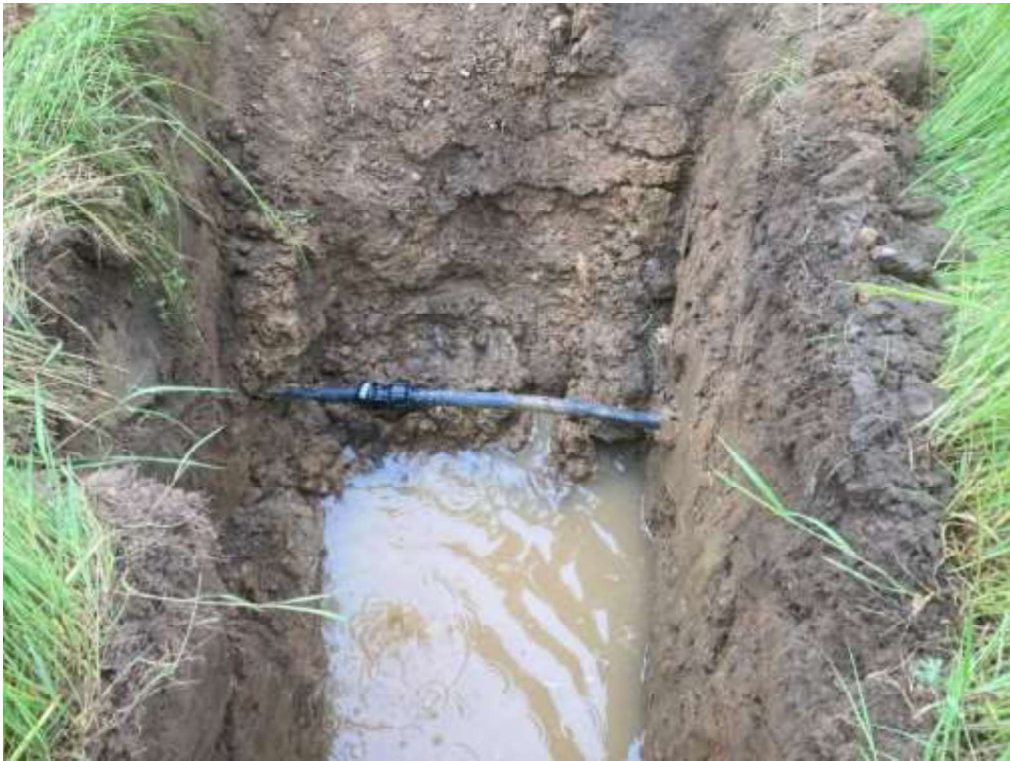
TP17 – Trial Pit
