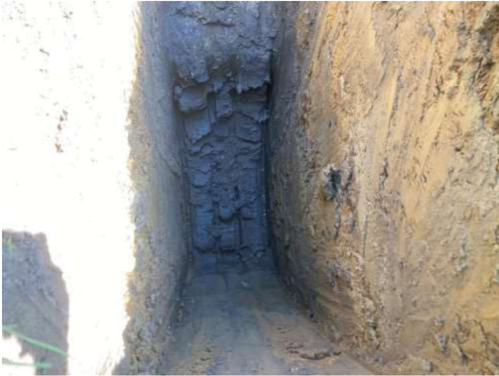
TP32 – Trial Pit
