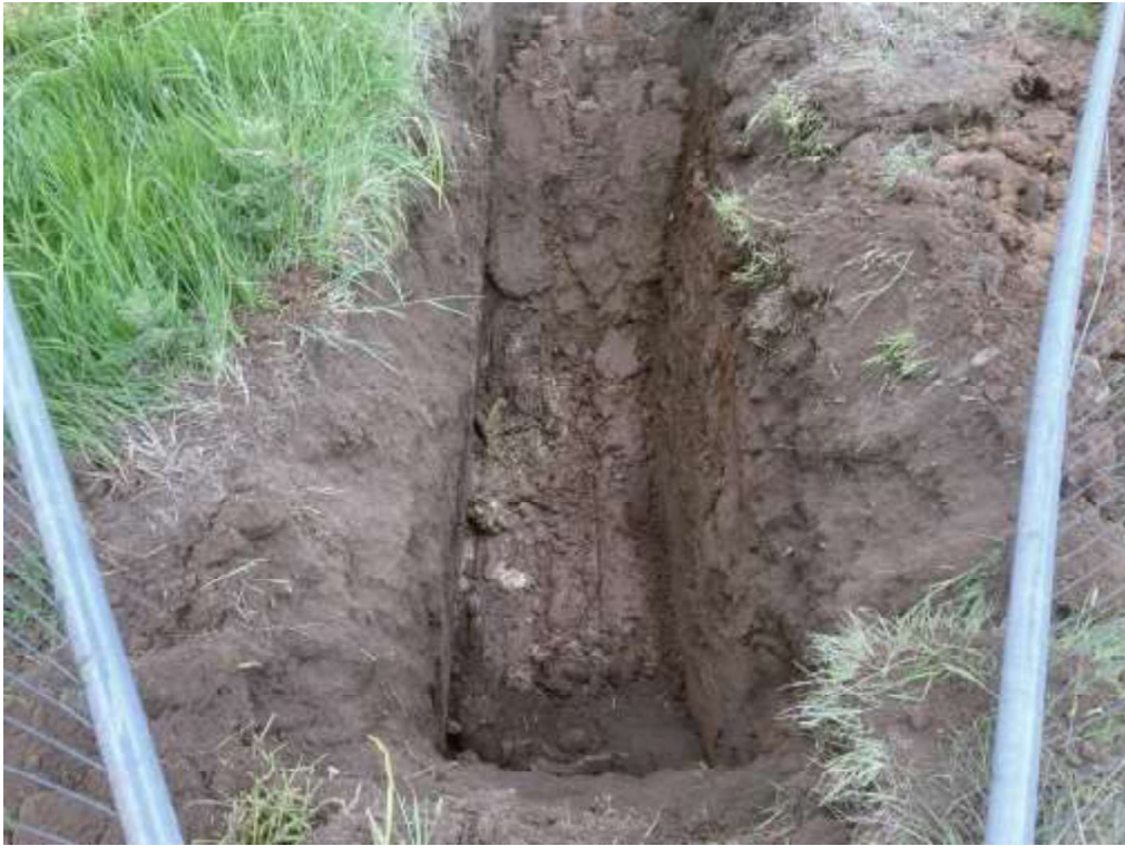
SA02 – Trial Pit
