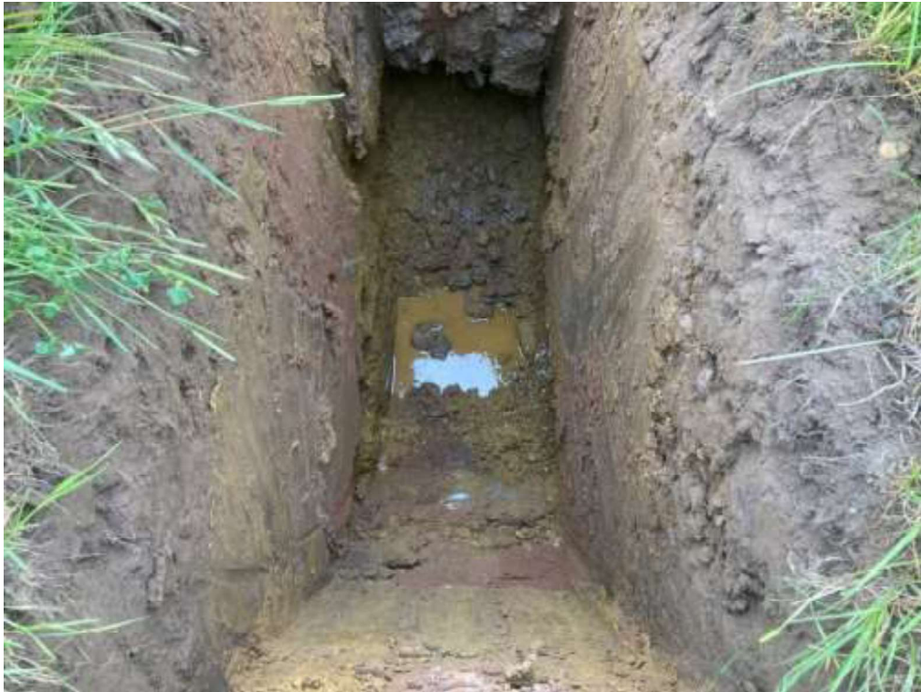
TP10 – Trial Pit
