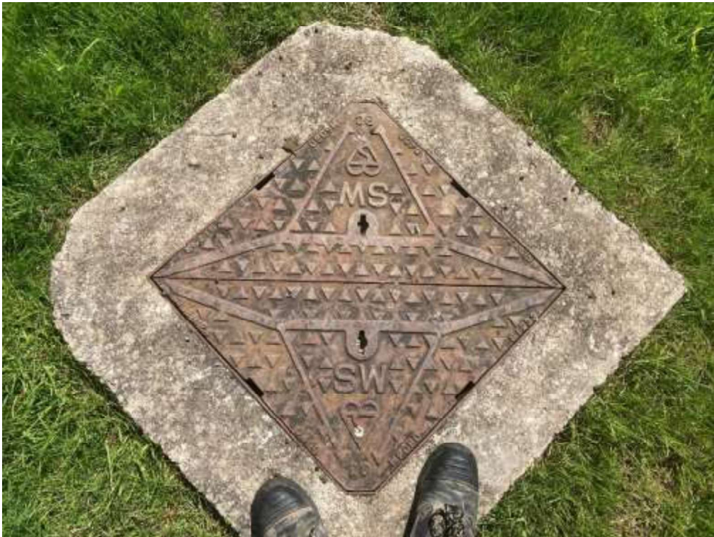
Looking down at a manhole cover on the eastern boundary
