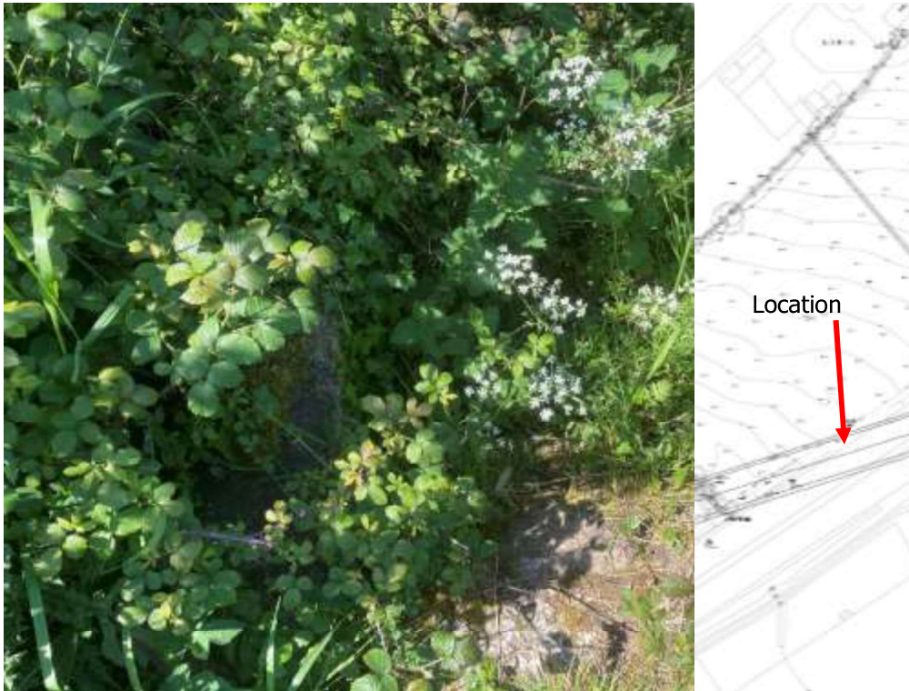
Looking west at a dry concrete drainage structure passing beneath the motorway
