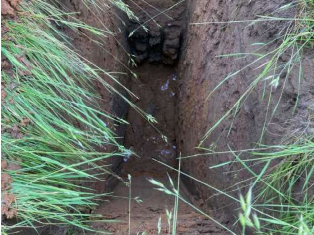
TP08 – Trial Pit
