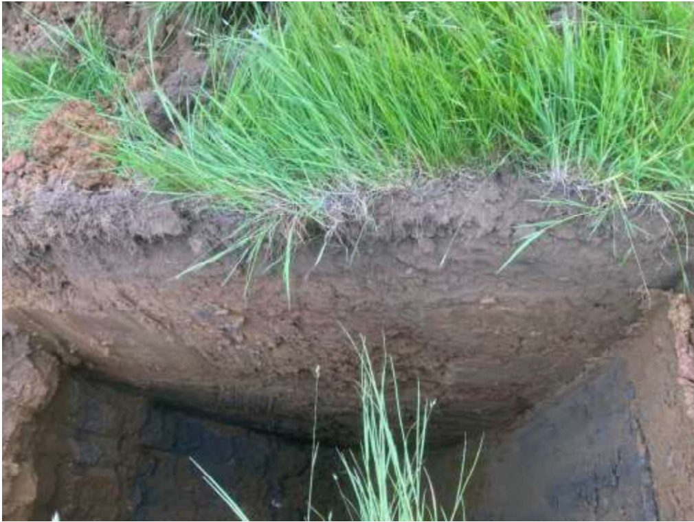
TP14 – Trial Pit
