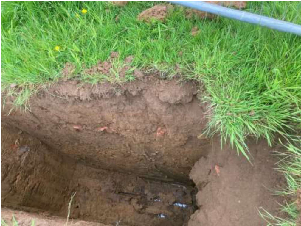
SA03 – Trial Pit
