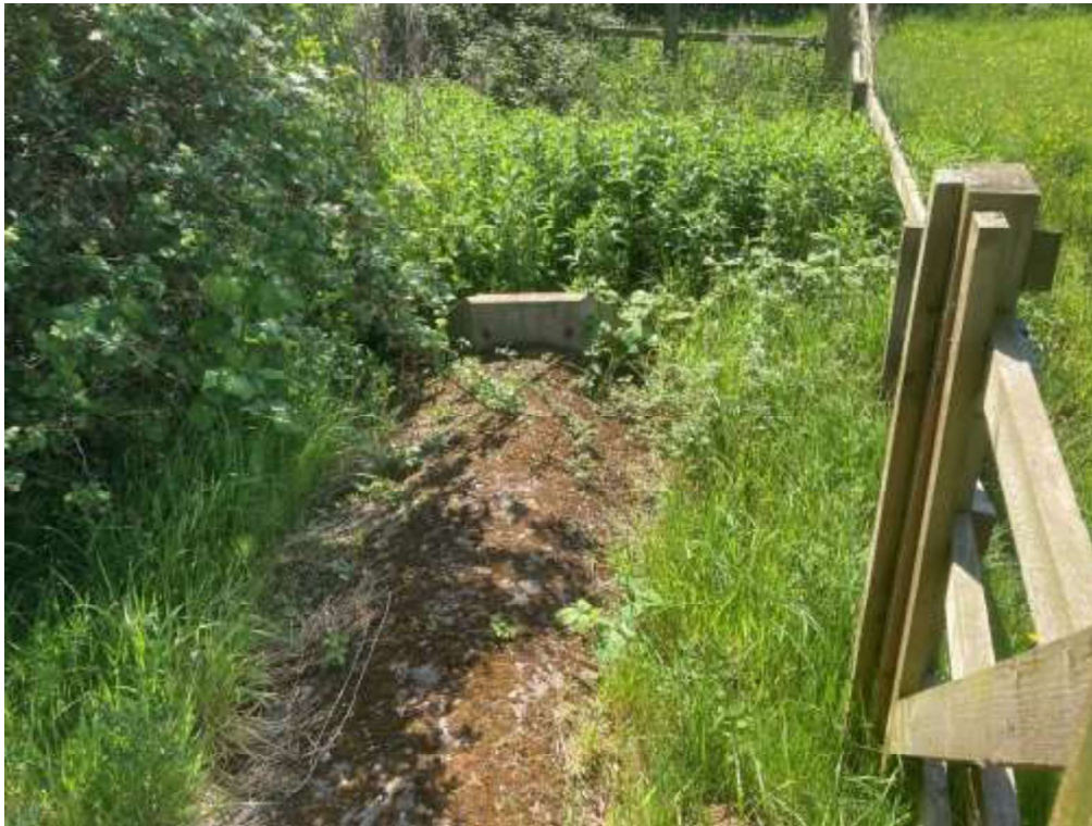
Looking south at the drainage outlet to the stream
