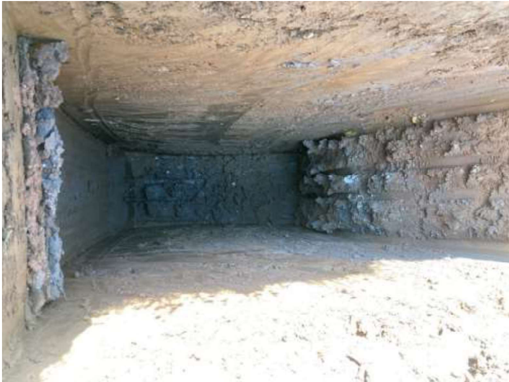
TP30 – Trial Pit
