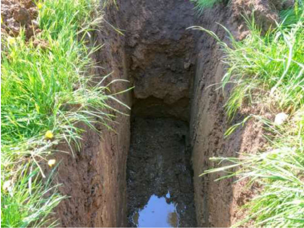
TP29 – Trial Pit
