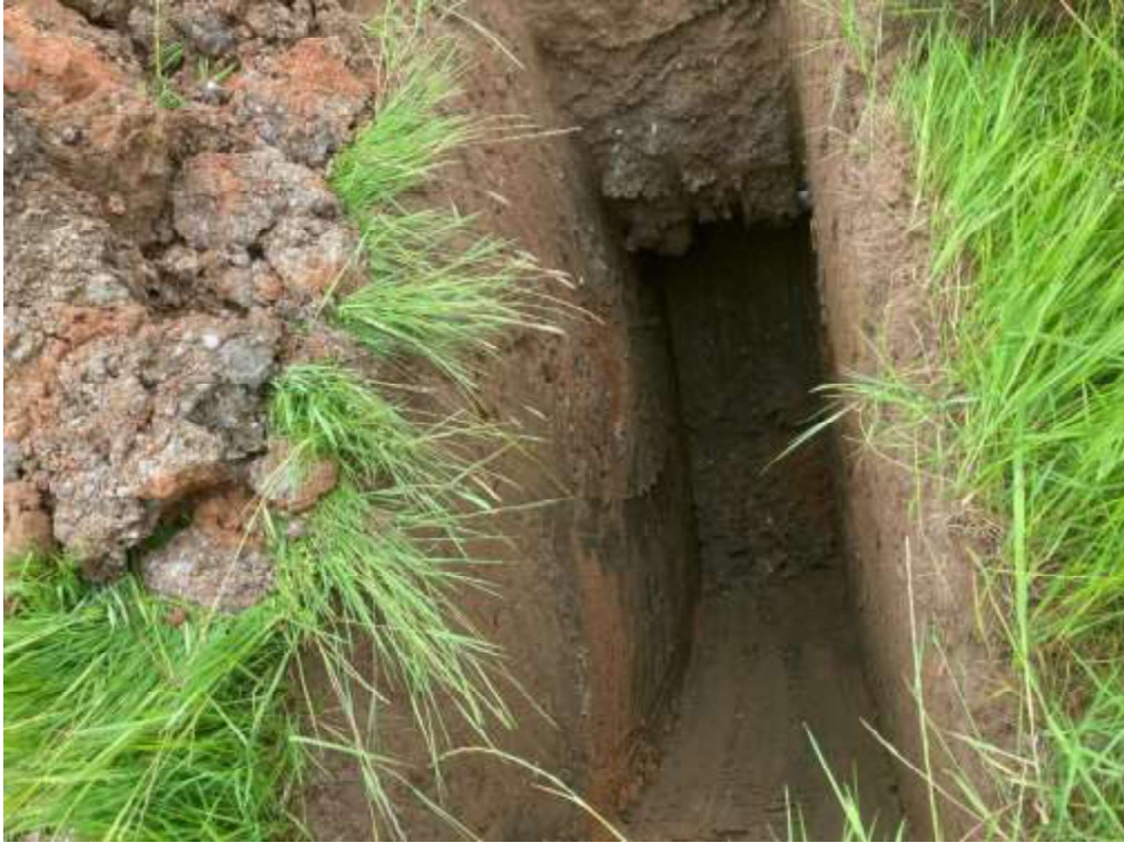
TP18 – Trial Pit
