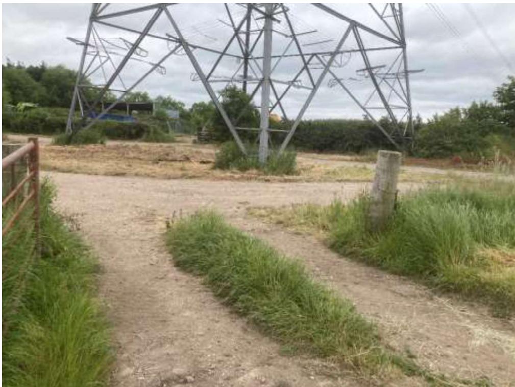
Showing the footprint of the electricity pylon at the end of Bullfurlong Lane
