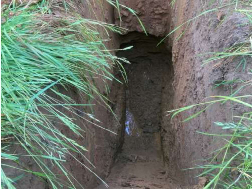
TP21 – Trial Pit
