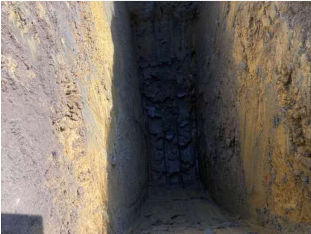
TP39 – Trial Pit
