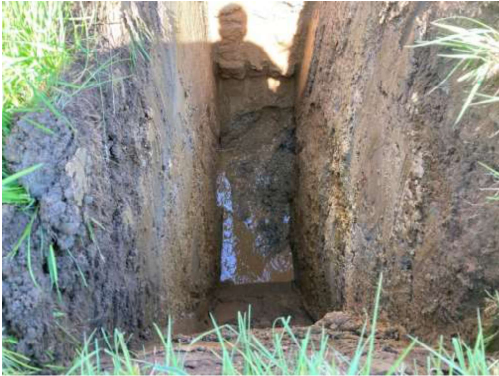
TP07 – Trial Pit
