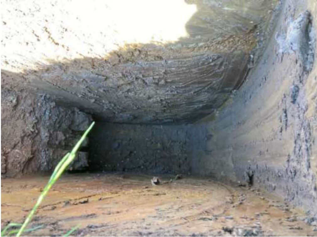
TP46 – Trial Pit
