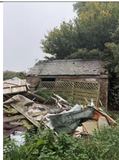
Plate 12. B4 as viewed from the south
