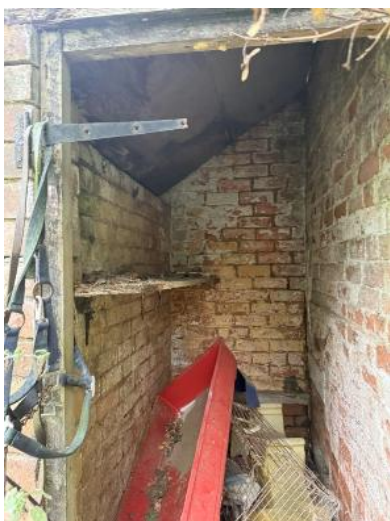
Plate 13. B4 internal view of eastern half of building
