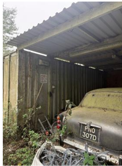
Plate 10. Connecting roof between B2a and B2b
