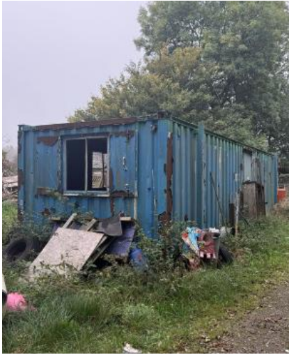
Plate 7. B1 as viewed from the south
