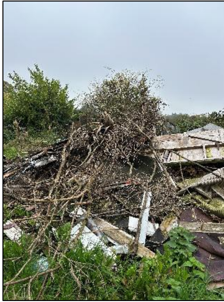
Plate 16. Debris pile on site (looking south)
