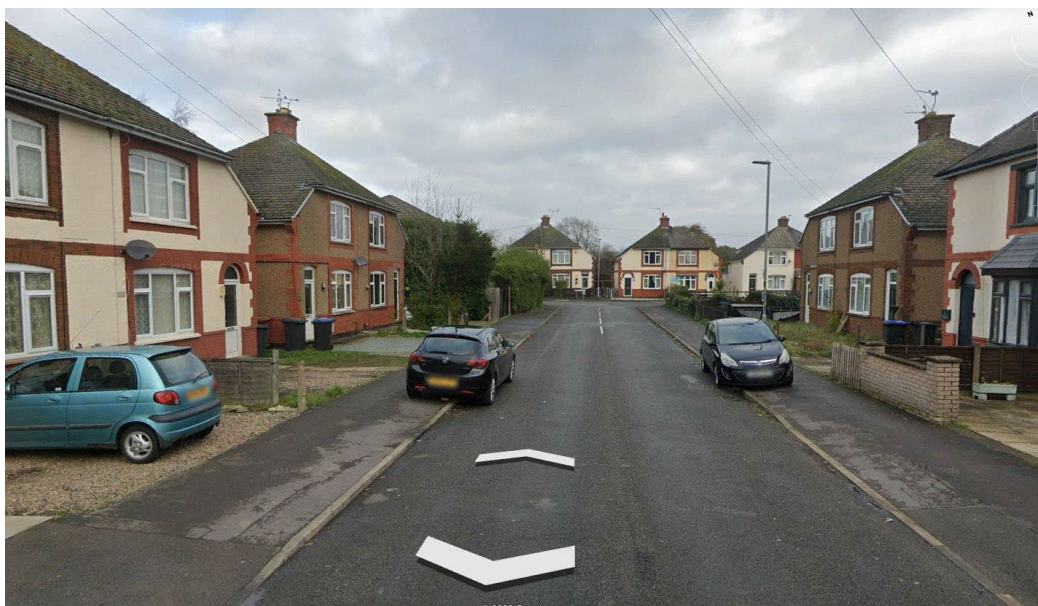
Figure 3.9: Example of current semi-detached housing stock in Barwell
