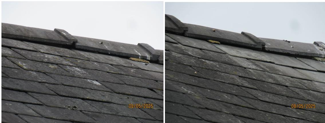
The verge can be repaired by leaving 2 50mm wide gaps, one on the north and one on the southern elevation, where there is no mortar between the slate and the solid brick wall. This will retain bat roosting for crevice dwelling bats in the building.
