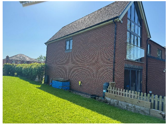
Figure 8: A-1.2 Developed land; sealed surface.
