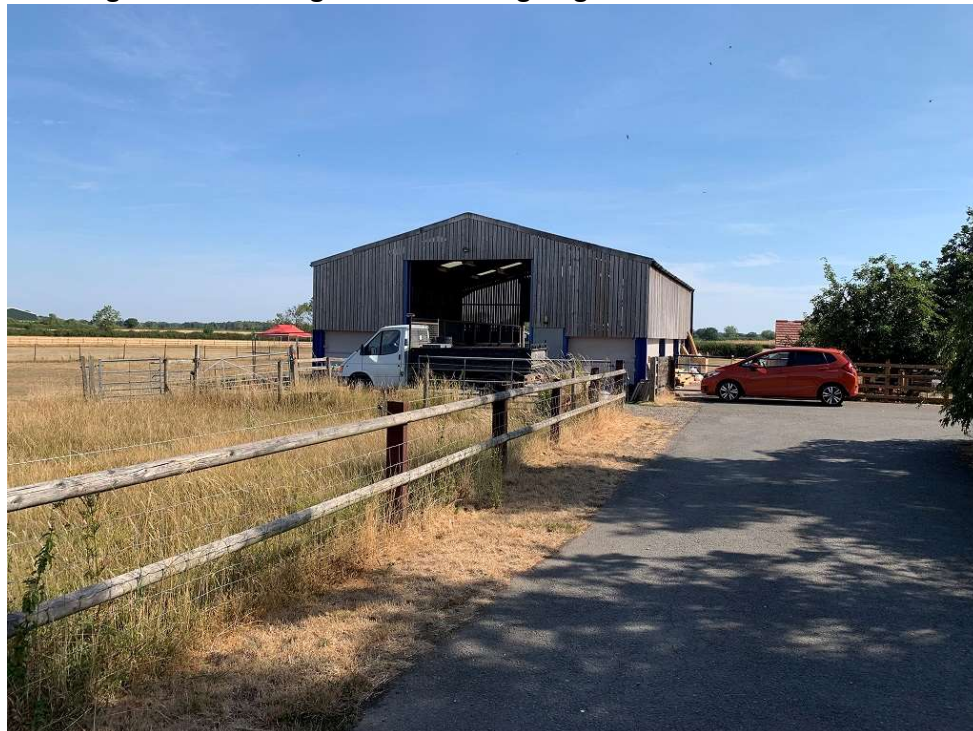
Figure 26: The barn to the north of the PDA, looking east
