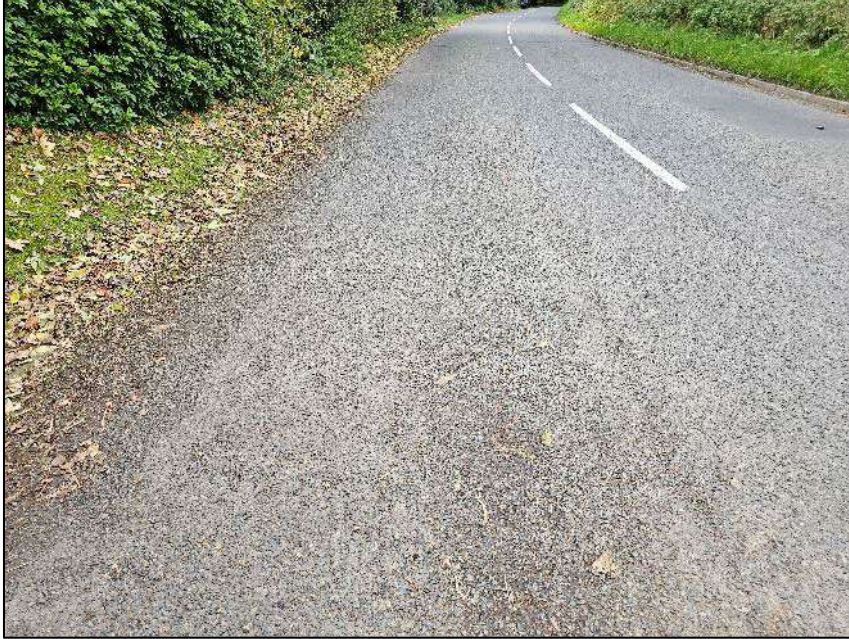
Figure 114: General Carriageway Condition 170m East of the Lychgate Lane Junction
