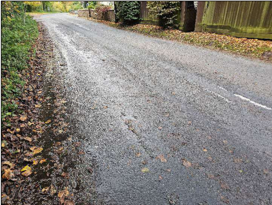
Figure 116: General Carriageway Condition 60-70m East of the Lychgate Lane Junction
