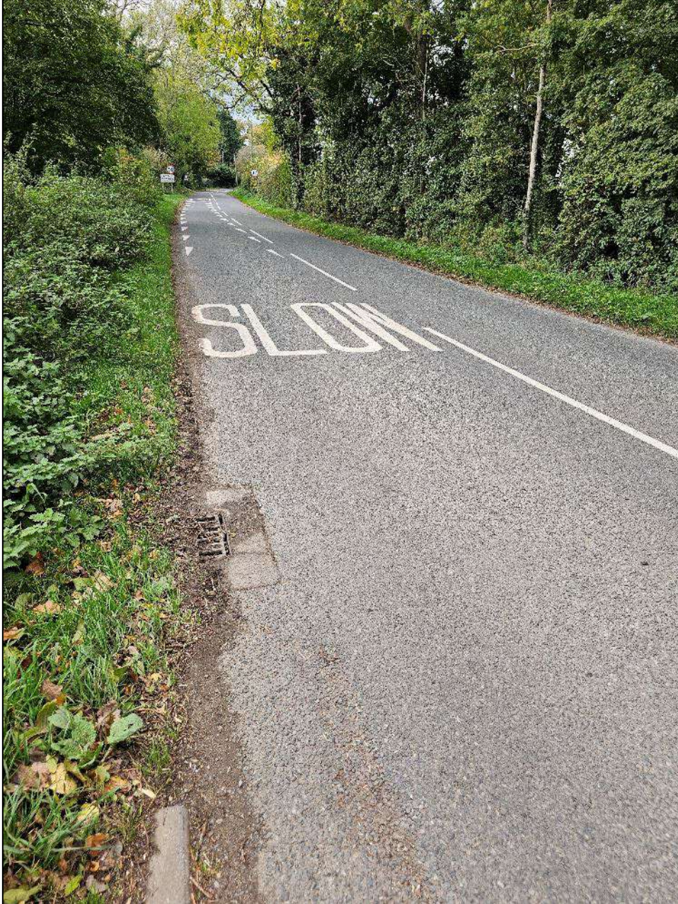
Figure 113: General Carriageway Condition 375m East of the Lychgate Lane Junction
