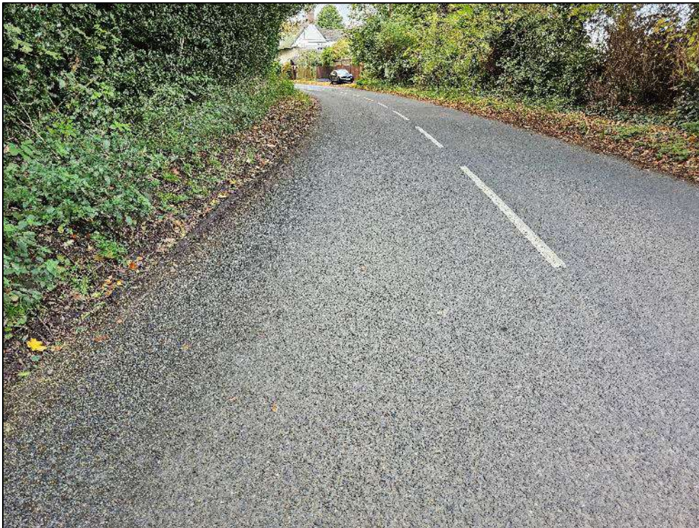
Figure 115: General Carriageway Condition 90m East of the Lychgate Lane Junction
