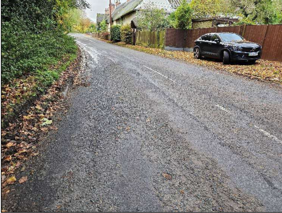
Figure 115: General Carriageway Condition 60-70m East of the Lychgate Lane Junction
