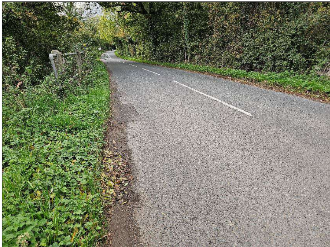
Figure 112: General Carriageway Condition 400m East of the Lychgate Lane Junction
