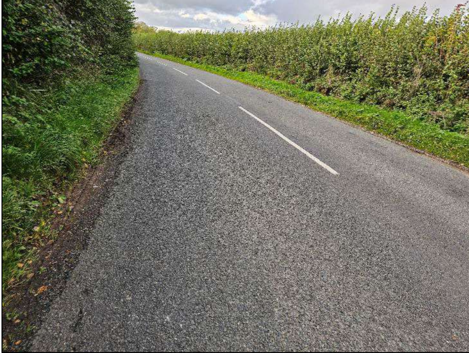
Figure 106: General Carriageway Condition 750m East of the Lychgate Lane Junction
