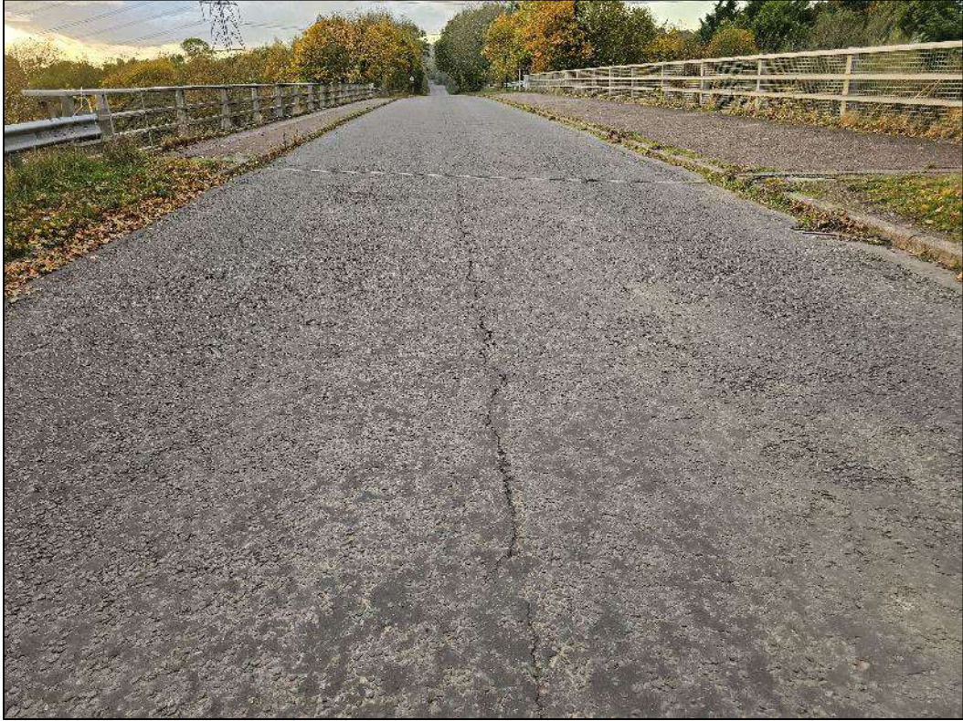
Figure 75: Surface Tarmac Transverse Cracks 160m East of the Parcel A Access
