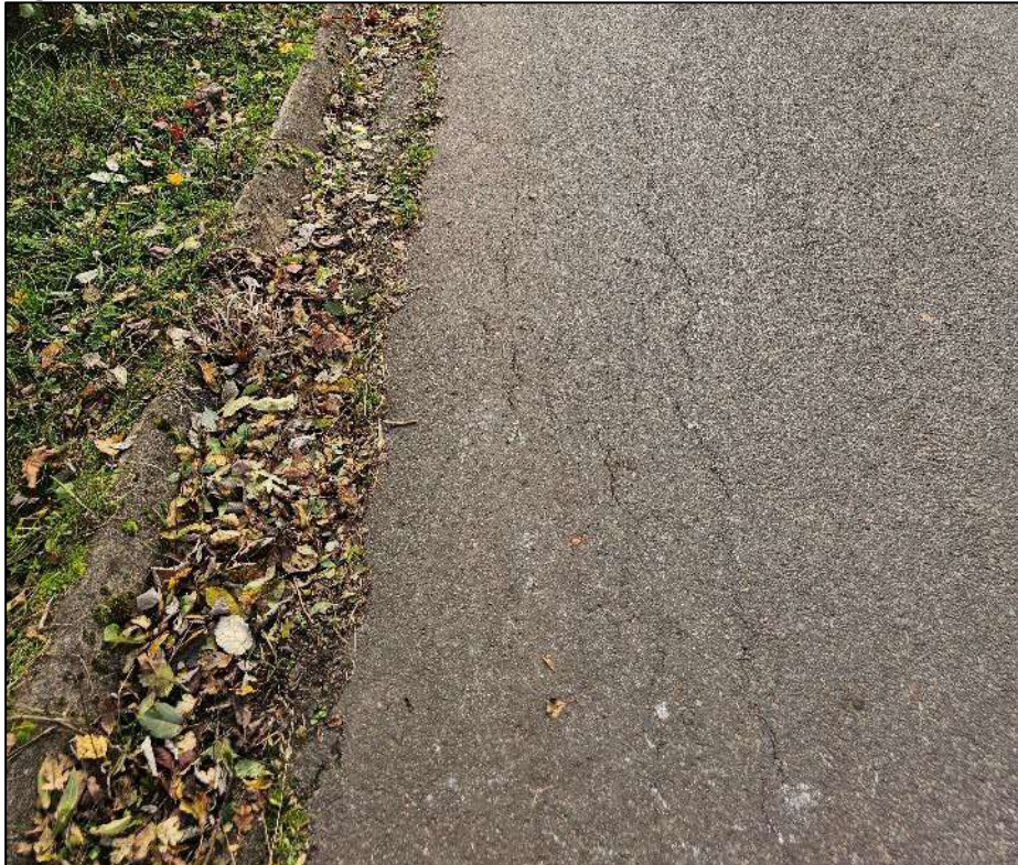
Figure 67: Tarmac Cracks 450m East of the Parcel A Access
