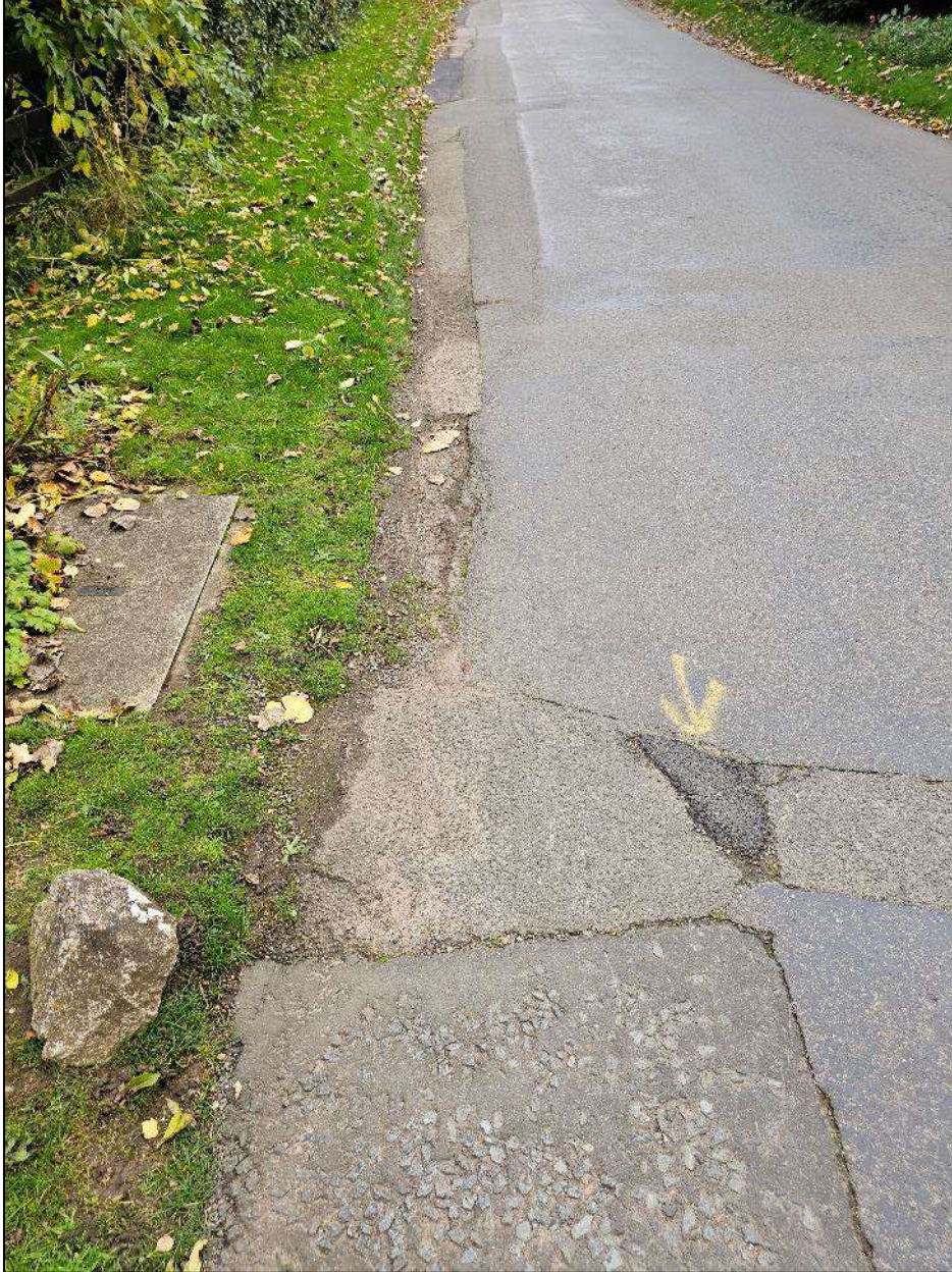
Figure 56: Carriageway Patching on Lychgate Lane, Approximately 900m East of the Parcel A Access
