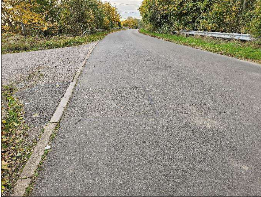
Figure 72: Debris Adjacent to Kerbing, and Tarmac Cracks 220-230m East of the Parcel A Access
