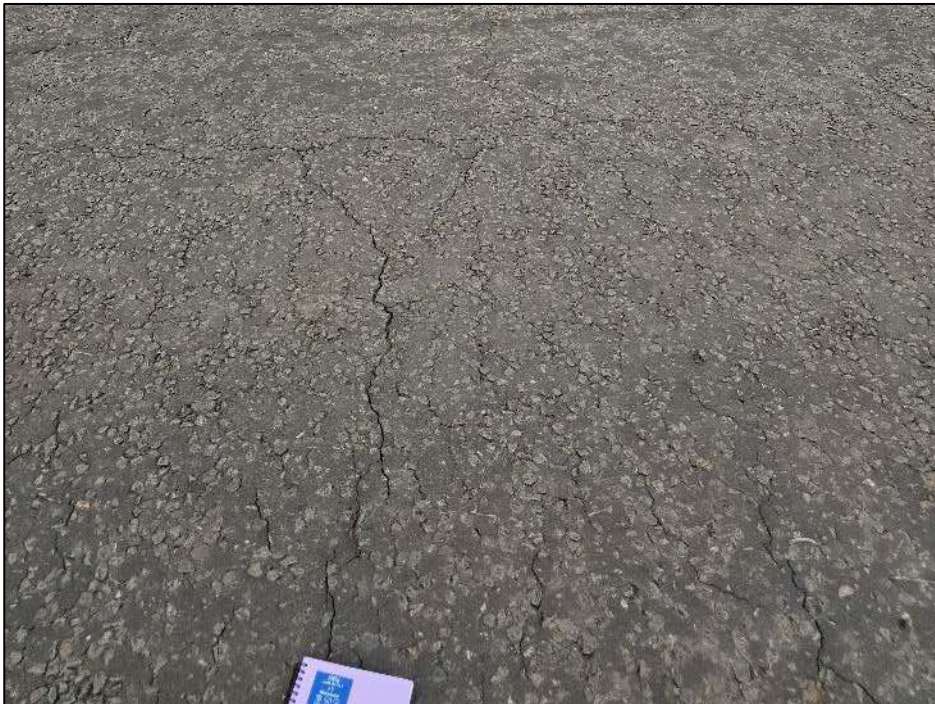
Figure 75: Surface Tarmac Transverse Cracks 160m East of the Parcel A Access
