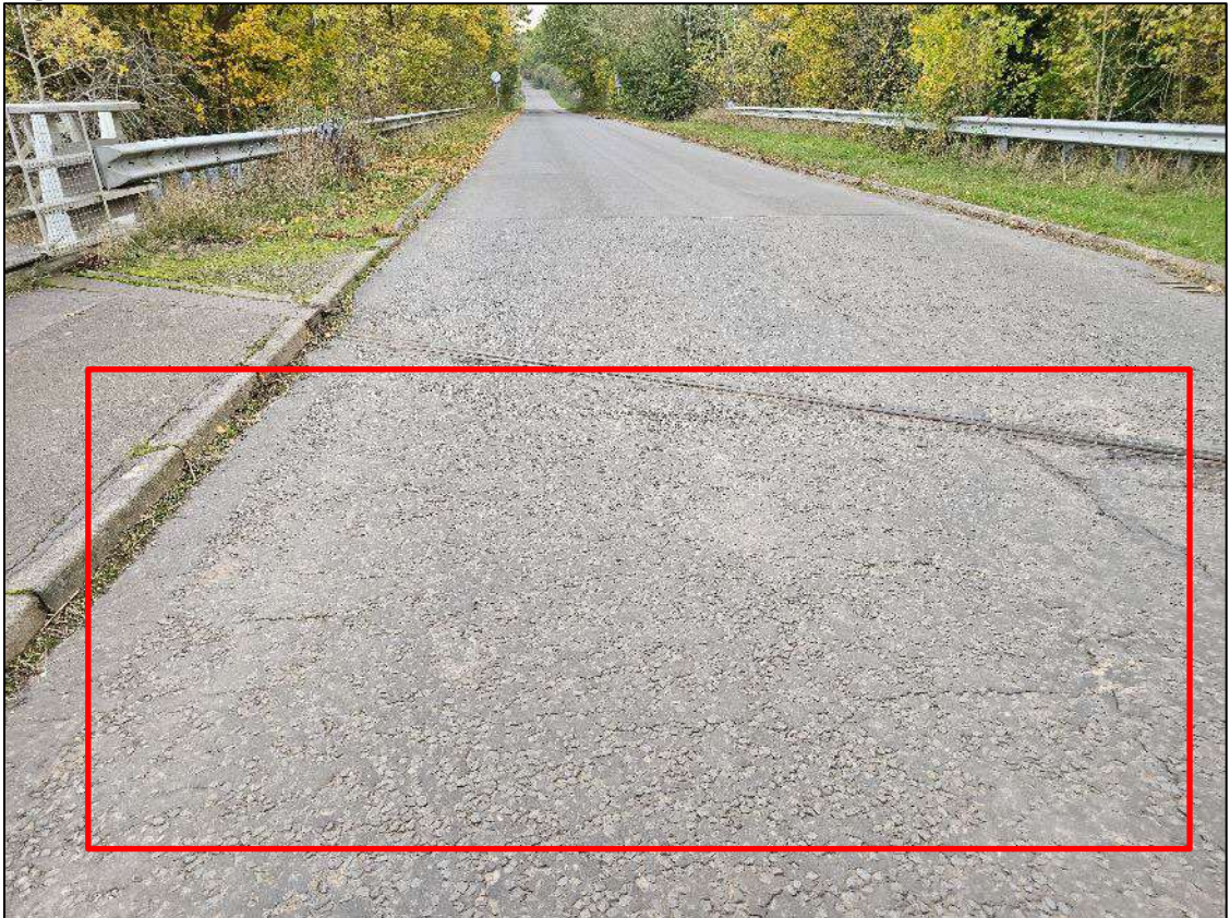
Figure 77: Transverse Surface Cracks 120m east of the Parcel A Access
