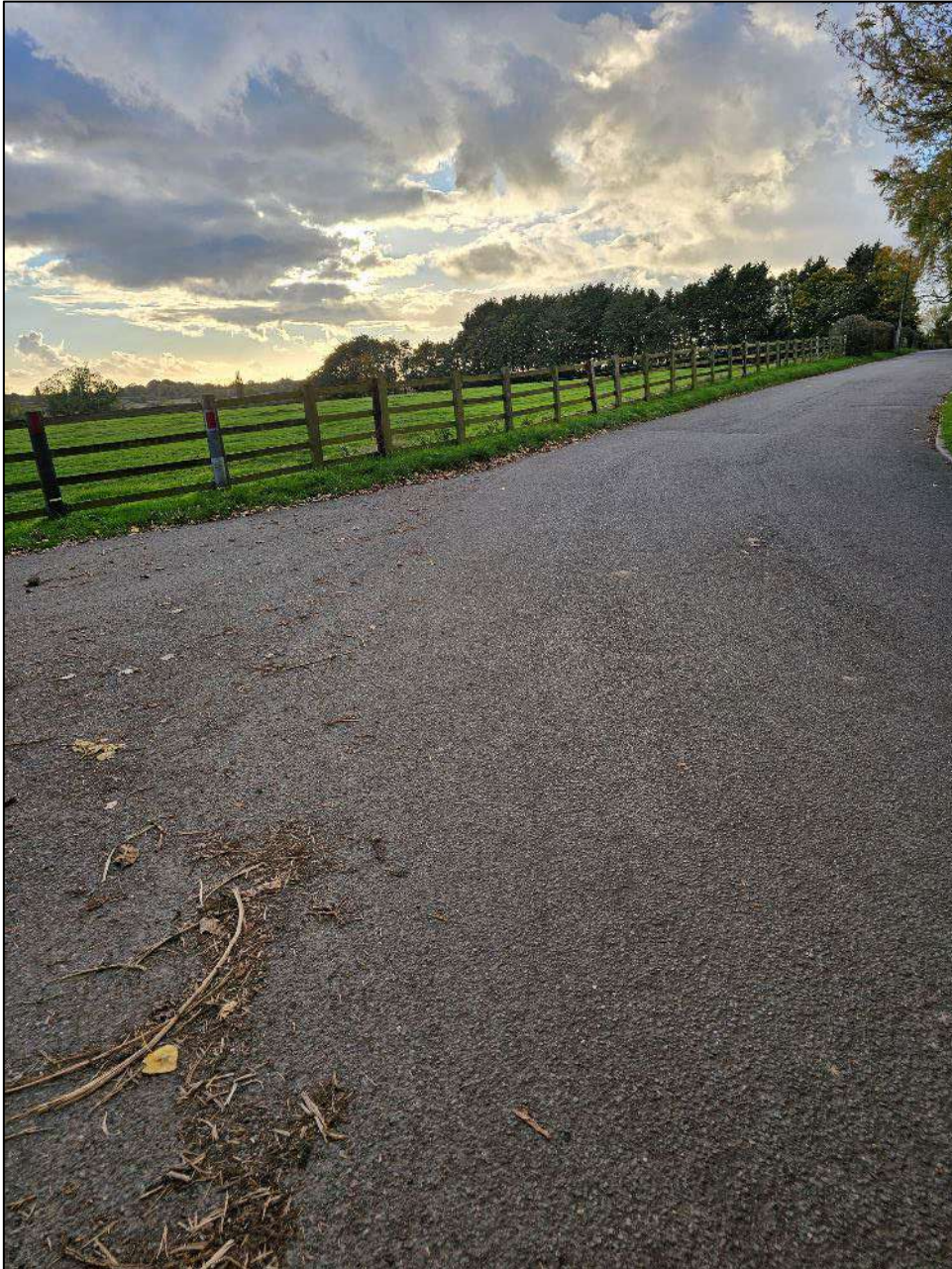
Figure 59: General Carriageway Condition at Lychgate Lane Bend
