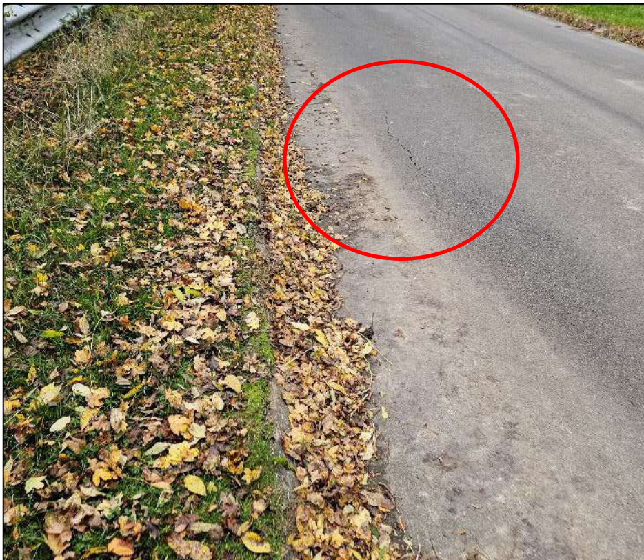
Figure 72: Debris Adjacent to Kerbing, and Tarmac Cracks 220-230m East of the Parcel A Access
