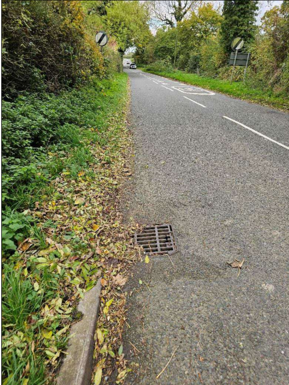
Figure 83: General Carriageway Condition 230-240m East of the Lychgate Lane Junction
