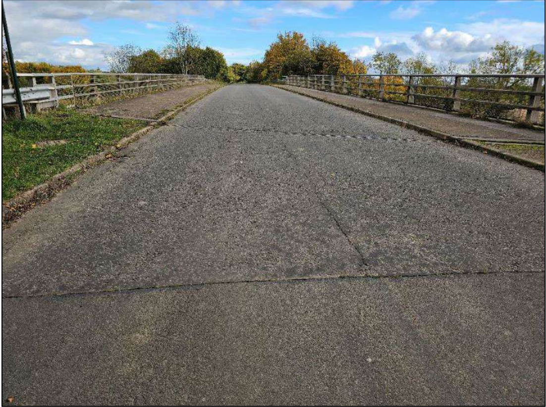
Figure 13: General Carriageway Condition 120m East of the Parcel A Access
