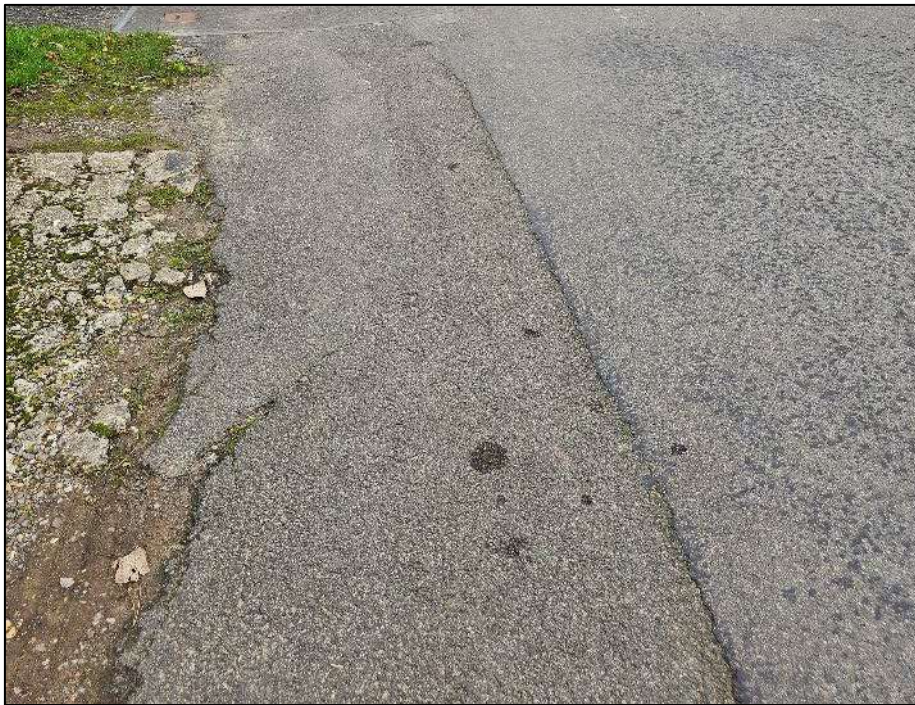
Figure 42: Carriageway Patching Approximately 950m East of the Parcel A Access
