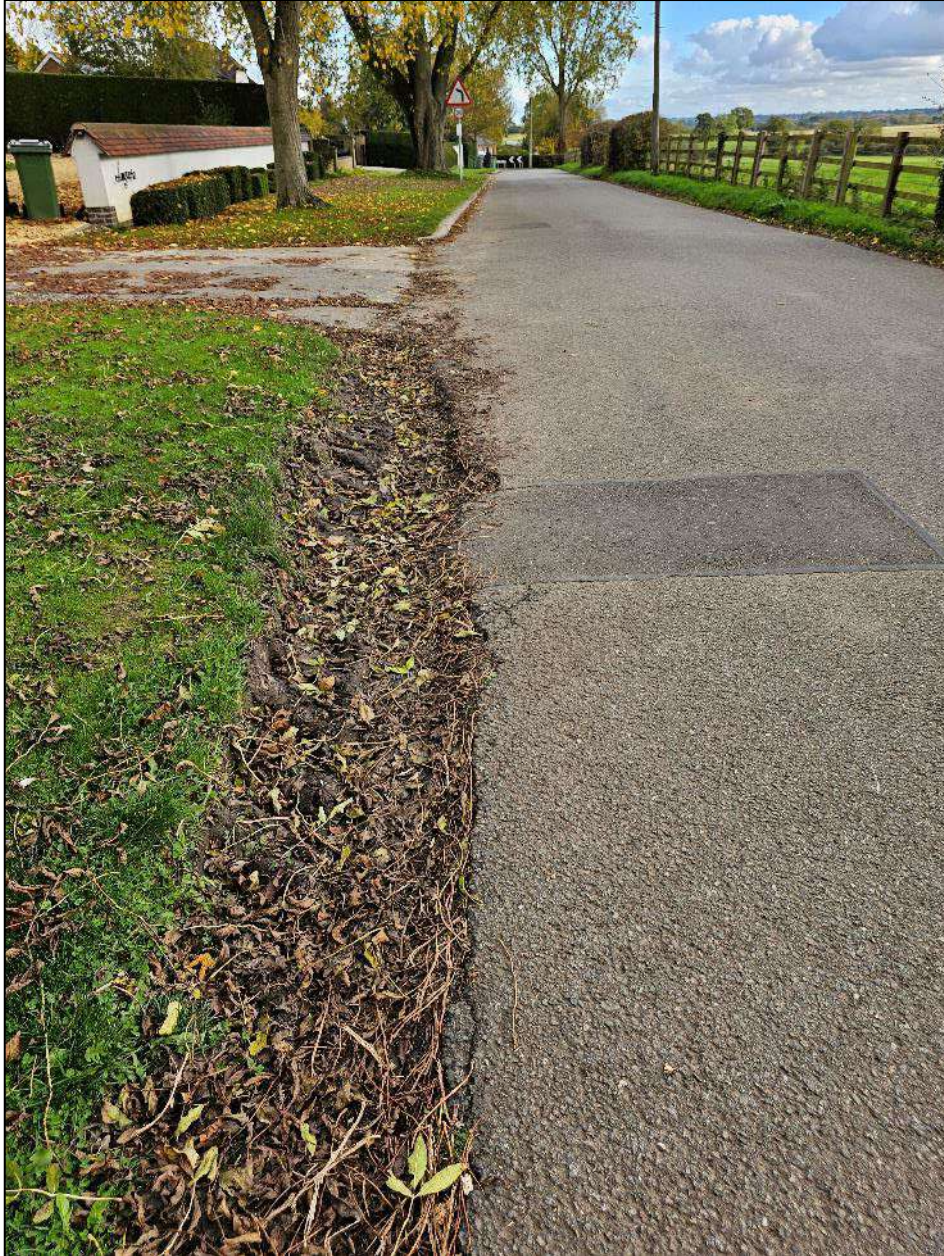
Figure 36: Grass Verge Damage Approximately 740m East of the Parcel A Access
