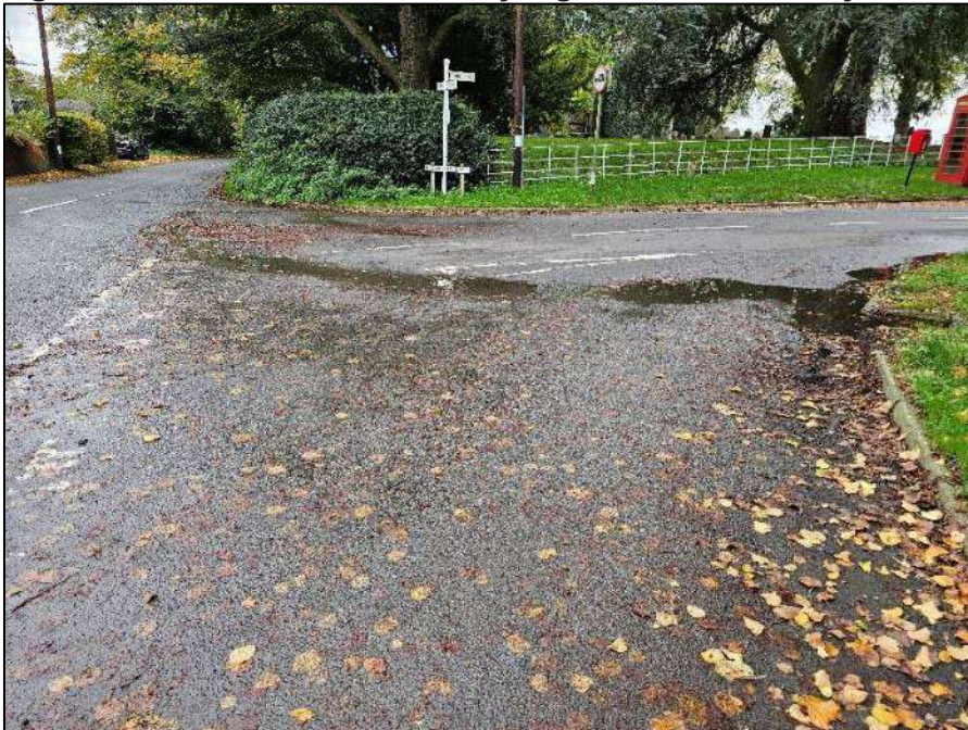
Figure 47: Blocked Drain at the Lychgate Lane / Hinckley Road Junction
