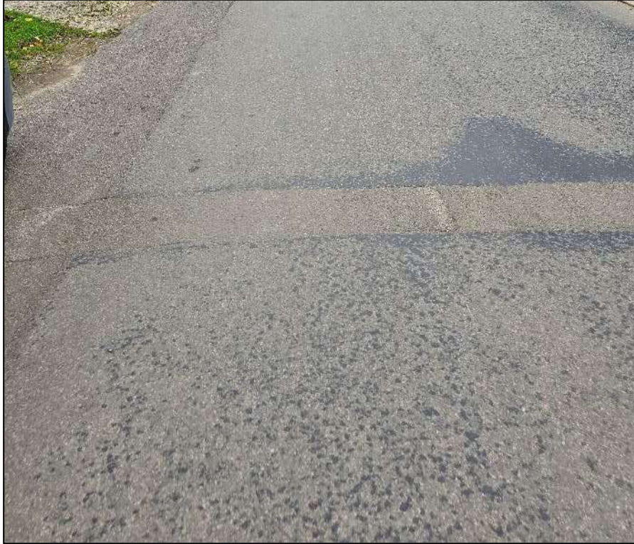
Figure 42: Carriageway Patching Approximately 950m East of the Parcel A Access
