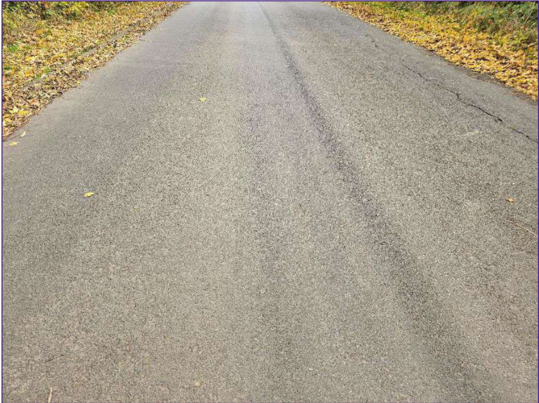
Figure 9: General Carriageway Condition 40m East of the Parcel A Access
