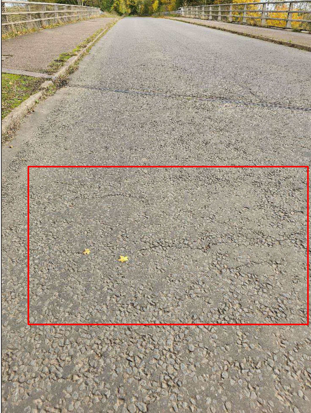
Figure 14: General Carriageway Condition 125m East of the Parcel A Access
