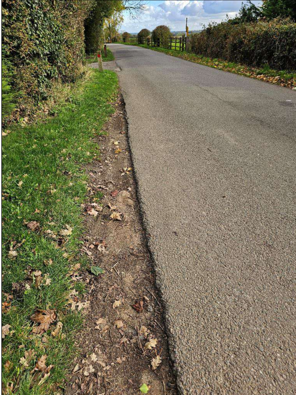
Figure 33: Grass Verge Degradation 650m East of the Parcel A Access
