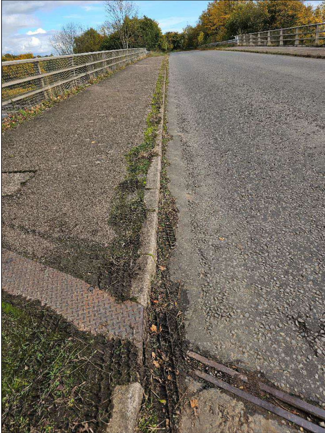
Figure 16: General Carriageway Condition 130m East of the Parcel A Access
