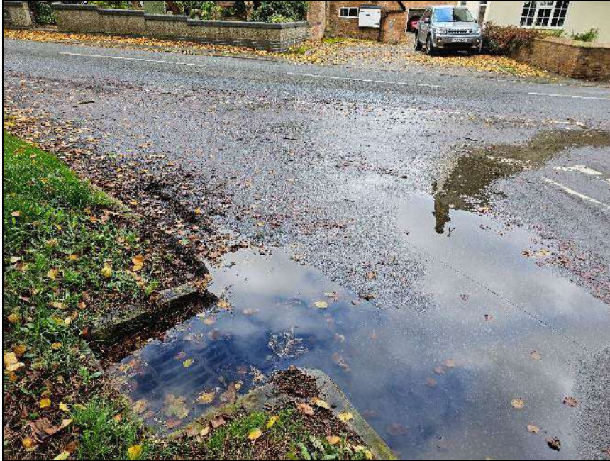
Figure 47: Blocked Drain at the Lychgate Lane / Hinckley Road Junction
