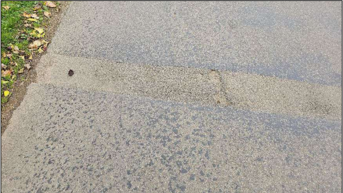
Figure 40: Carriageway Patching Approximately 930-940m East of the Parcel A Access
