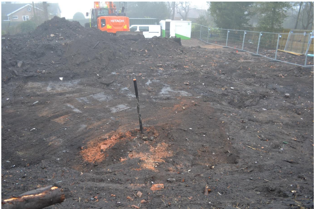
8: The site following ground reduction showing quarry backfill deposits
