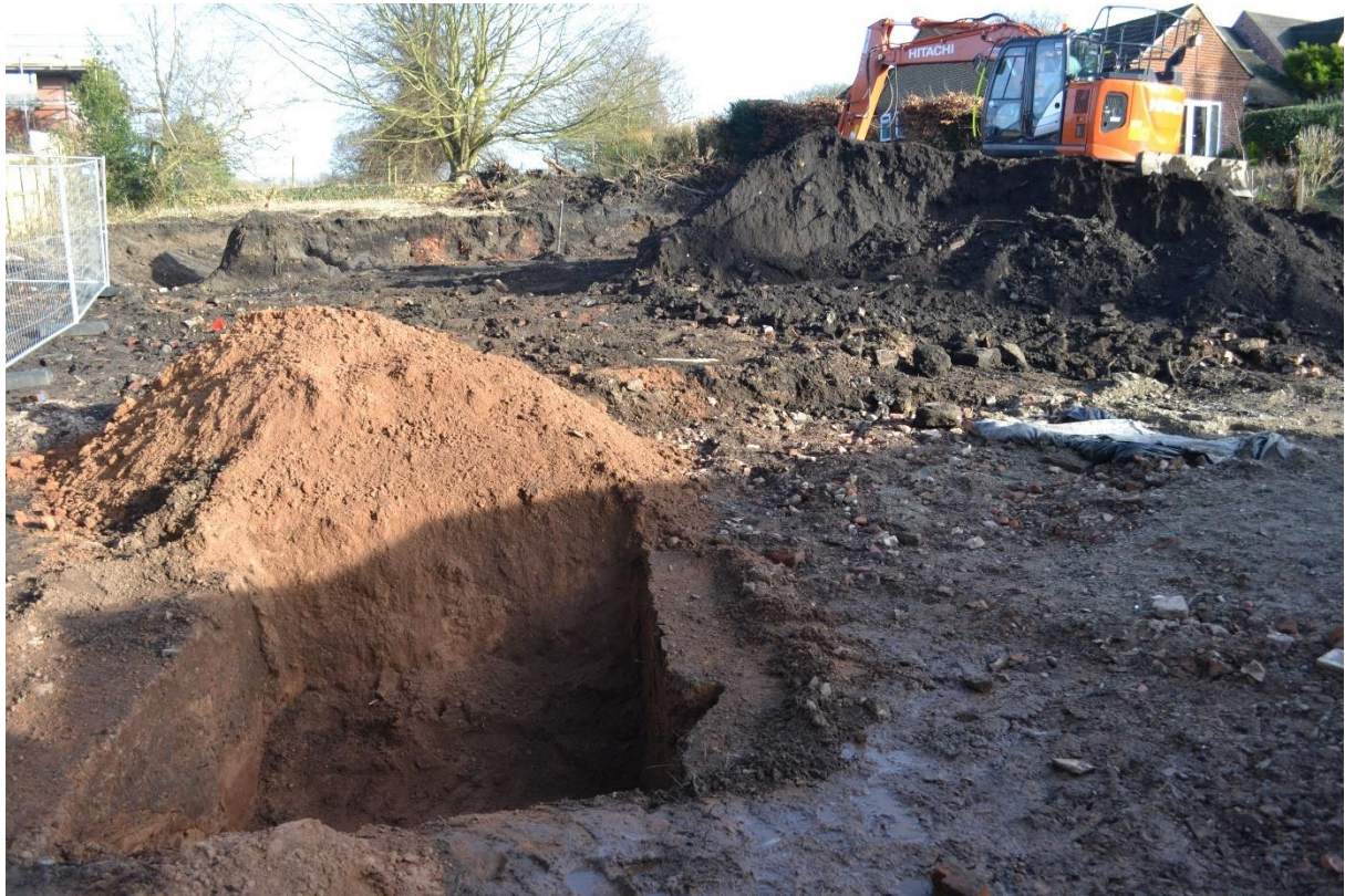
5: View east across site following excavation of sondage
