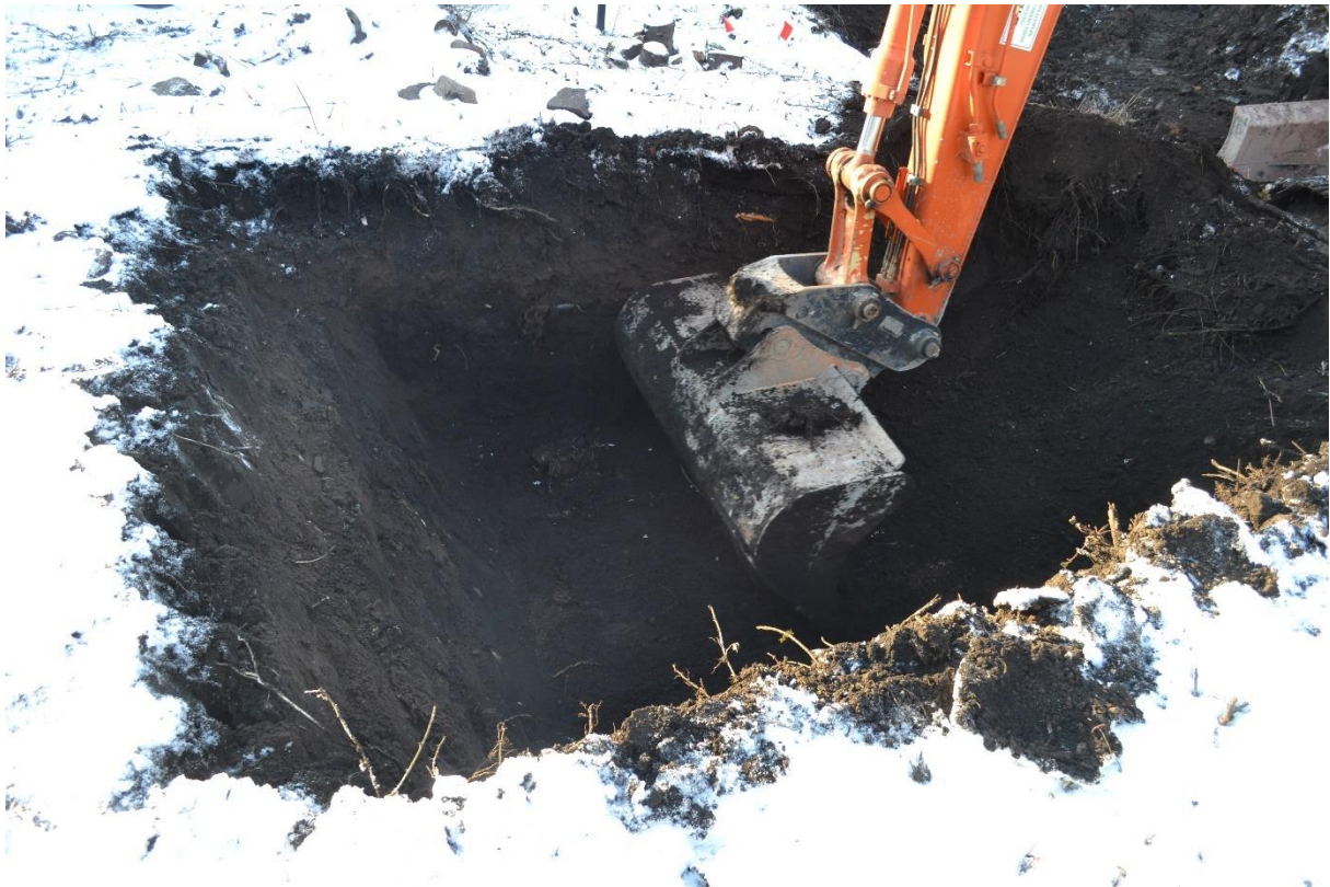
6: Machine excavation into quarry backfill deposits, looking SSW
