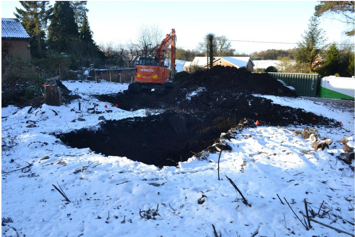
1: View south-west across site at start of works
