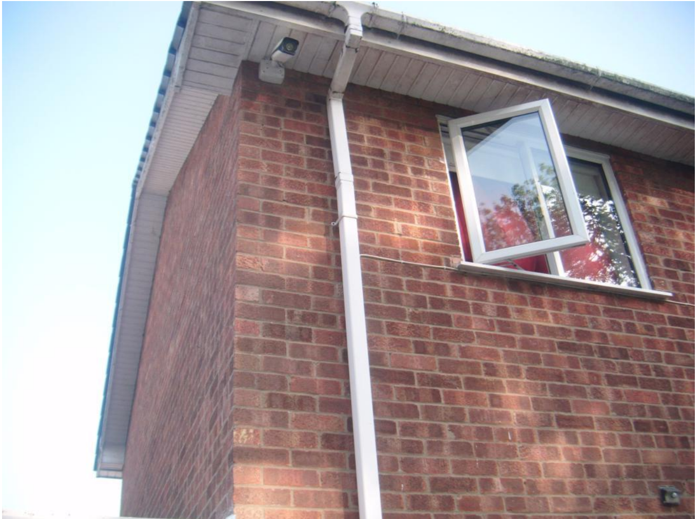
Rear soffit detail
