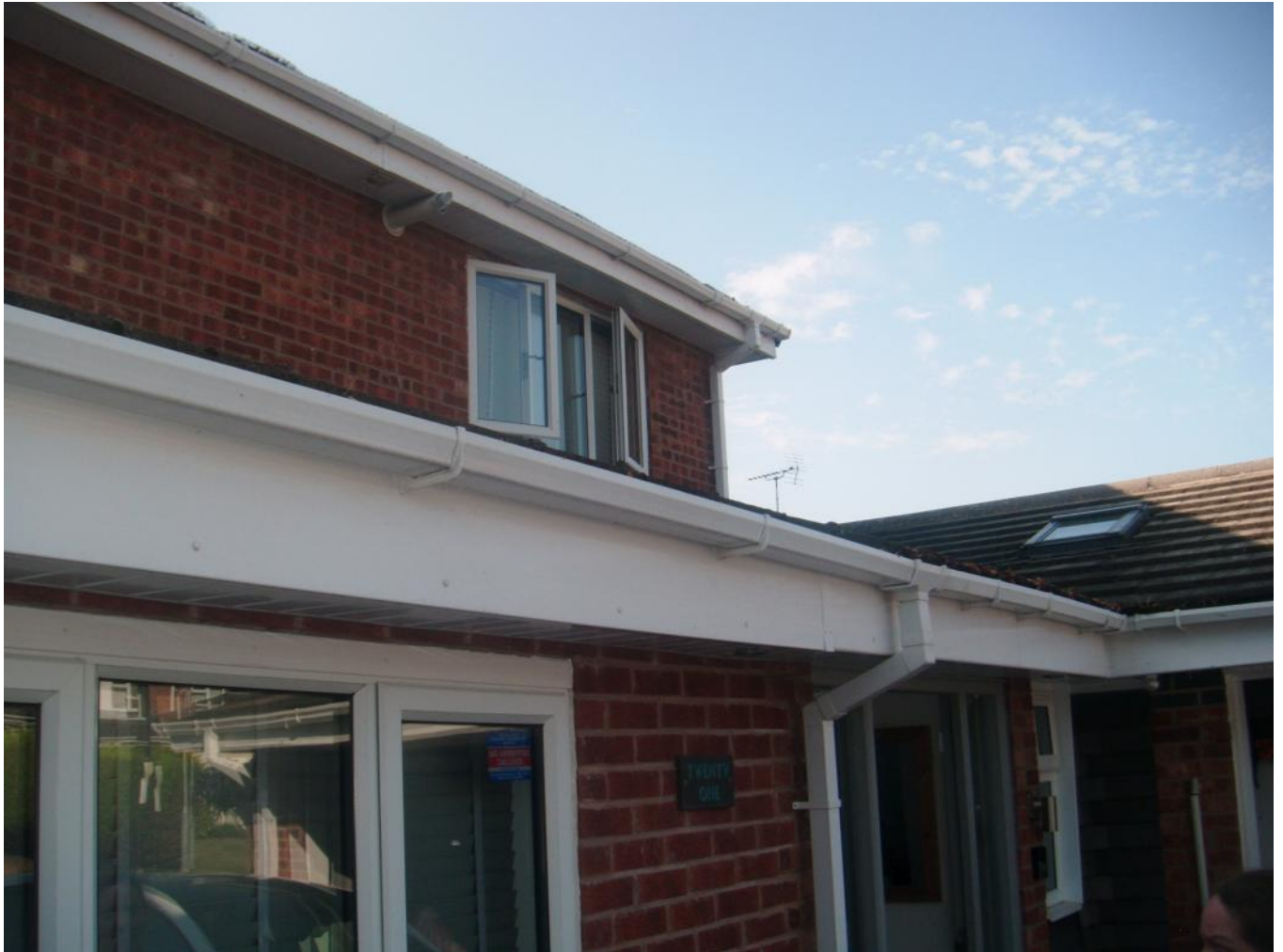
Front porch, UPVC clad soffits
