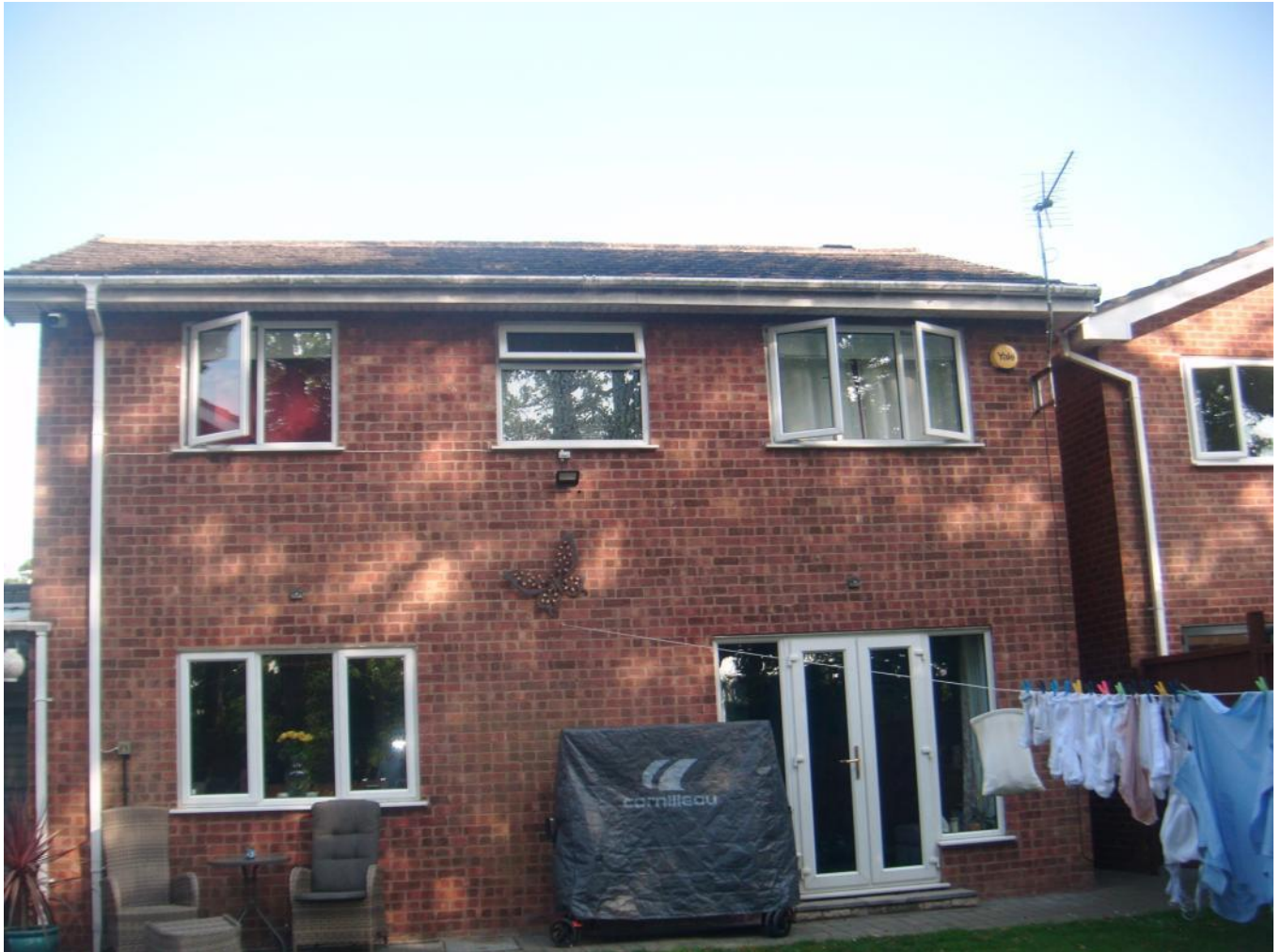
Rear showing roof
