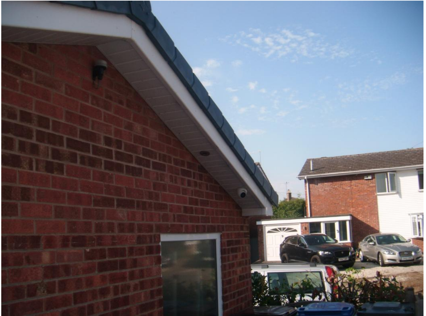
End: tight fitting UPVC
