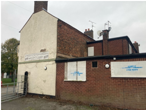
Plates 12-13: Photographs of the side and rear elevations of the Oddfellows, November 2024. These photographs show the historic rear elevation of the building with exposed brickwork and dentiled eaves brick detailing, alongside 20 th century single and two-storey extensions which do not contribute to its architectural value and/or aesthetic appeal. Removal of later additions and the concrete parking area would be a positive intervention.
