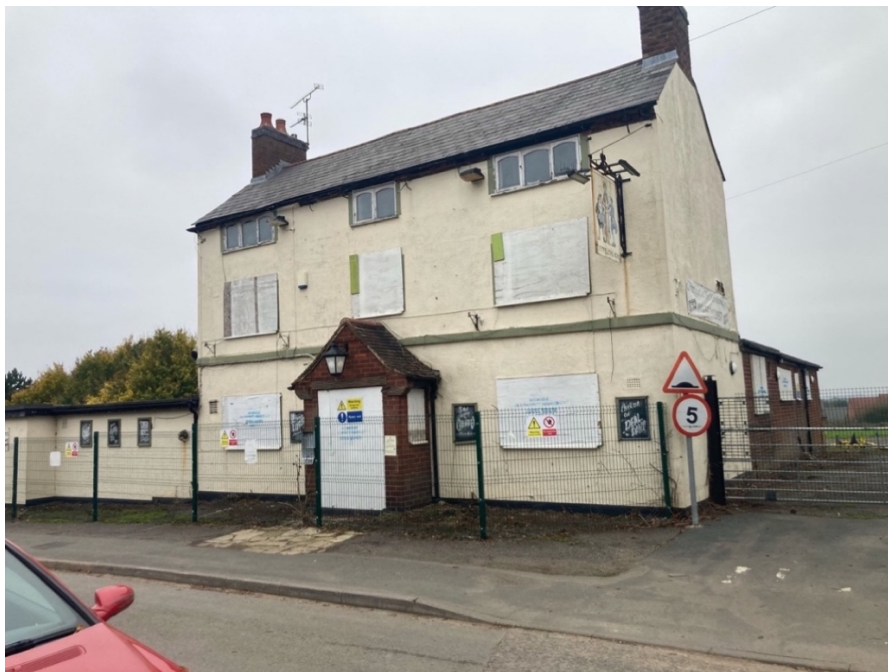
Plate 10: Photograph of the front elevation of the building, November 2024
