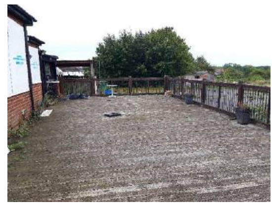
Rear Decked External Seating Area
