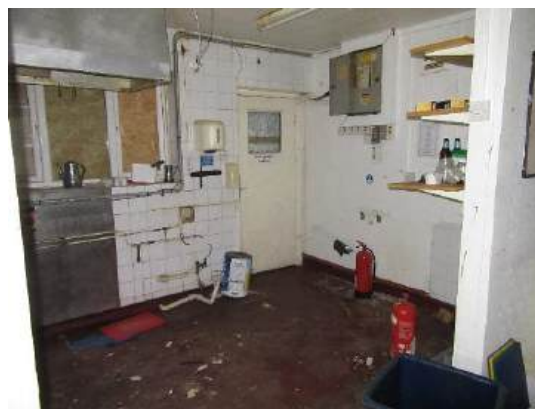
Former Commercial Kitchen
