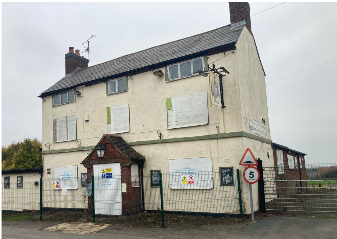
Plate 7: Photograph of the front and side elevation of the Oddfellows looking north, November 2024.
