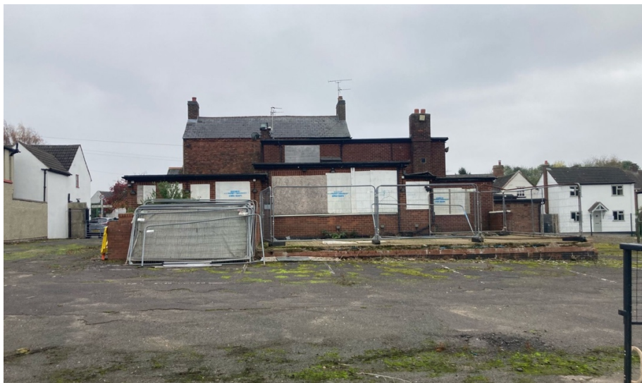
Plate 3: Photograph of the rear elevation of the Oddfellows Arms, November 2024
