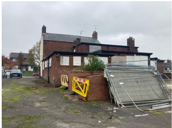
Plates 12-13: Photographs of the side and rear elevations of the Oddfellows, November 2024. These photographs show the historic rear elevation of the building with exposed brickwork and dentiled eaves brick detailing, alongside 20 th century single and two-storey extensions which do not contribute to its architectural value and/or aesthetic appeal. Removal of later additions and the concrete parking area would be a positive intervention.
