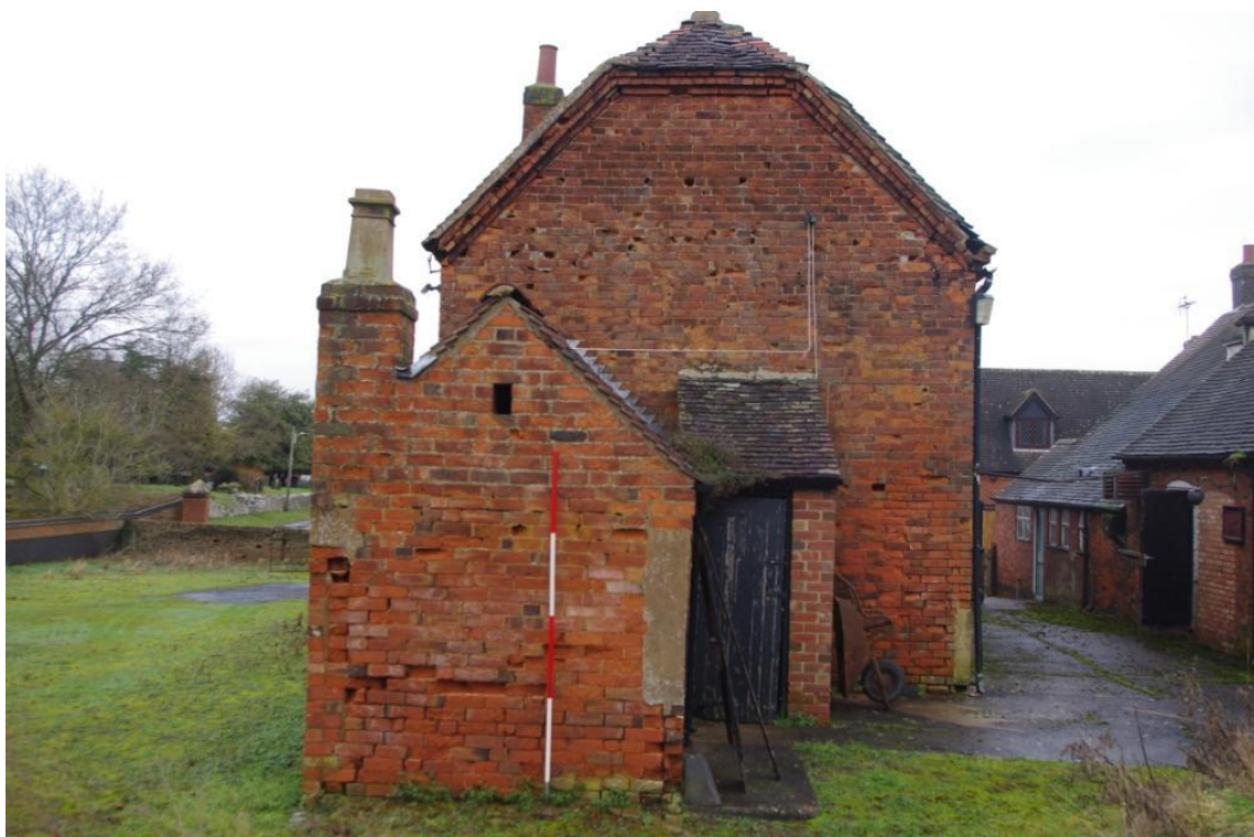
Figure 19 Building B, West – South West Facing Gable (Looking East – North East).
