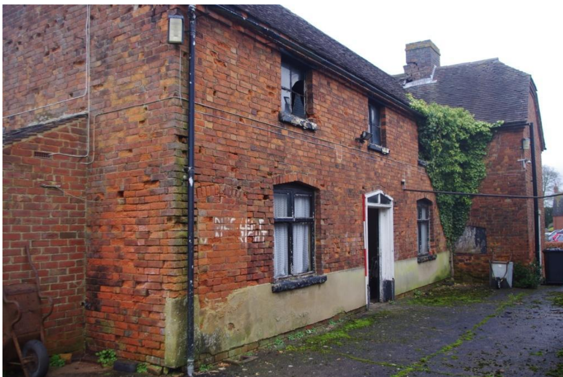
Figure 18 Building B, South – South East Facing Elevation (Looking North East).
