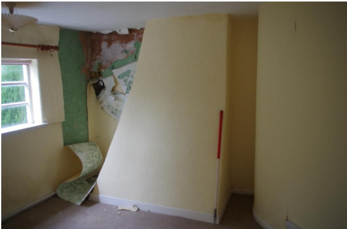
Figure 15 A (9), Chimney Breast (Looking West – South West).
