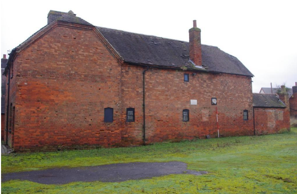
Figure 17 Building B , North – North West Facing Elevation (Looking South West).
