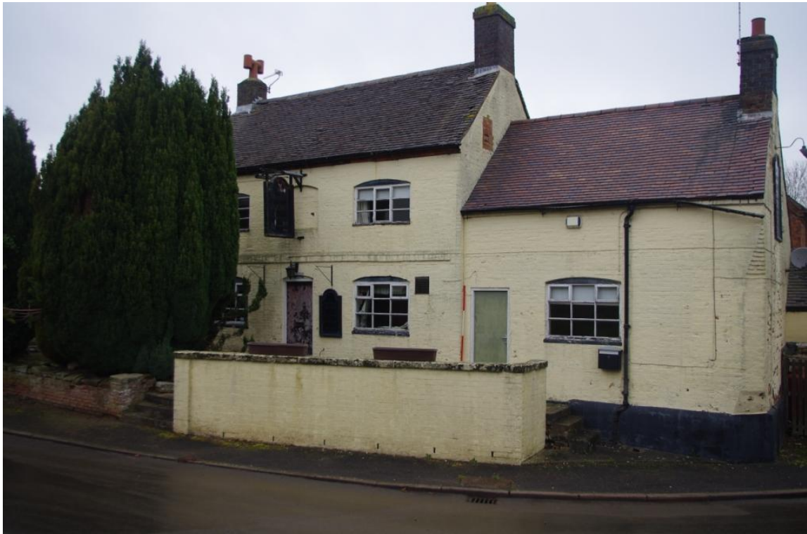
Figure 6 Building A , Principal Elevation (Looking North West).
