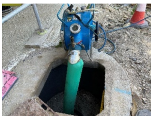
DRAIN LINING REPAIRS
