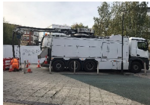
HIGH PRESSURE JETTING
