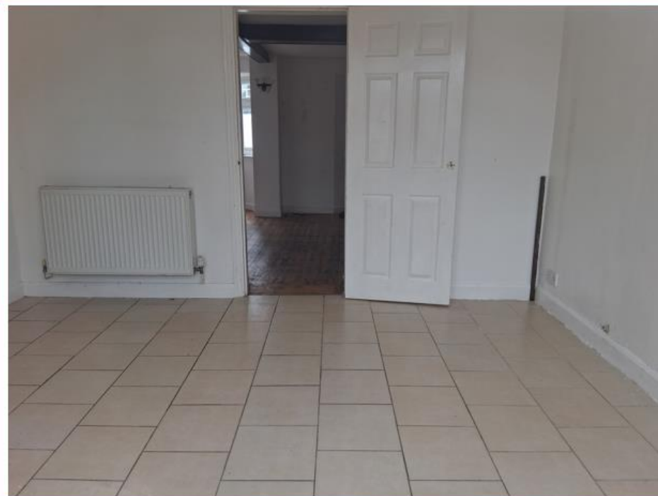
Photo No.22: Example shot of the interior of the disused dwelling, taken from outside the structure
