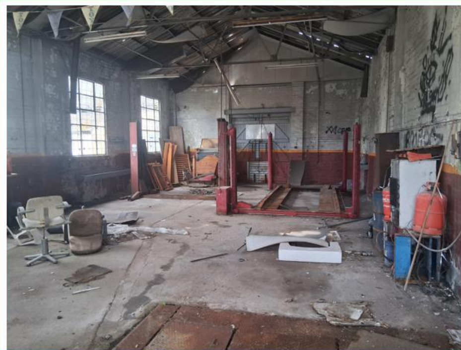
Photo No.34: Example shot of the interior of the former vehicle workshop forming the central extent of site
