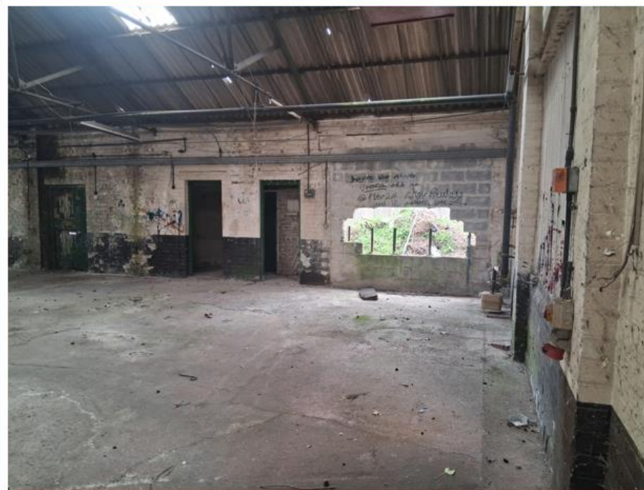
Photo No.16: Facing west from the far NE extent of eastern-most structure on site (back towards northern yard area)
