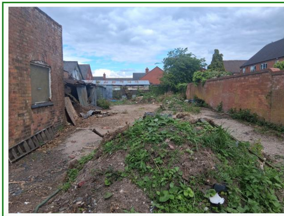
Photo No.26: Facing east showing the remaining southern exterior area on site (workshop to left) & further heaps
