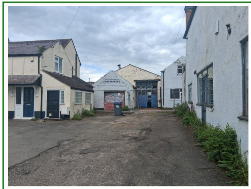
Photo No.24: Facing east from the SW extent of site showing the forecourt to workshops forming southern and eastern extents
