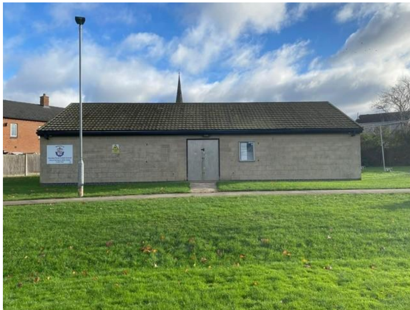
View looking south-east of existing front elevation – Hinckley Road Cricket Pavilion
