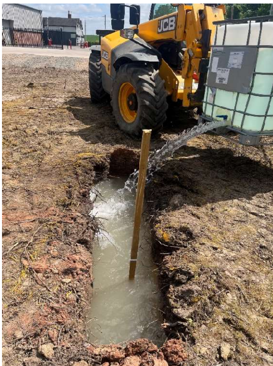
Figure 4: filling of test hole to 100% depth
