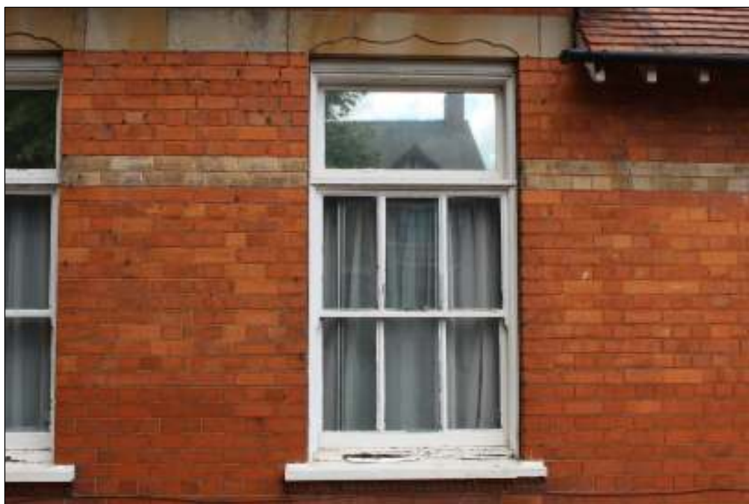
Photo 15 Sash window to the south facing elevation
