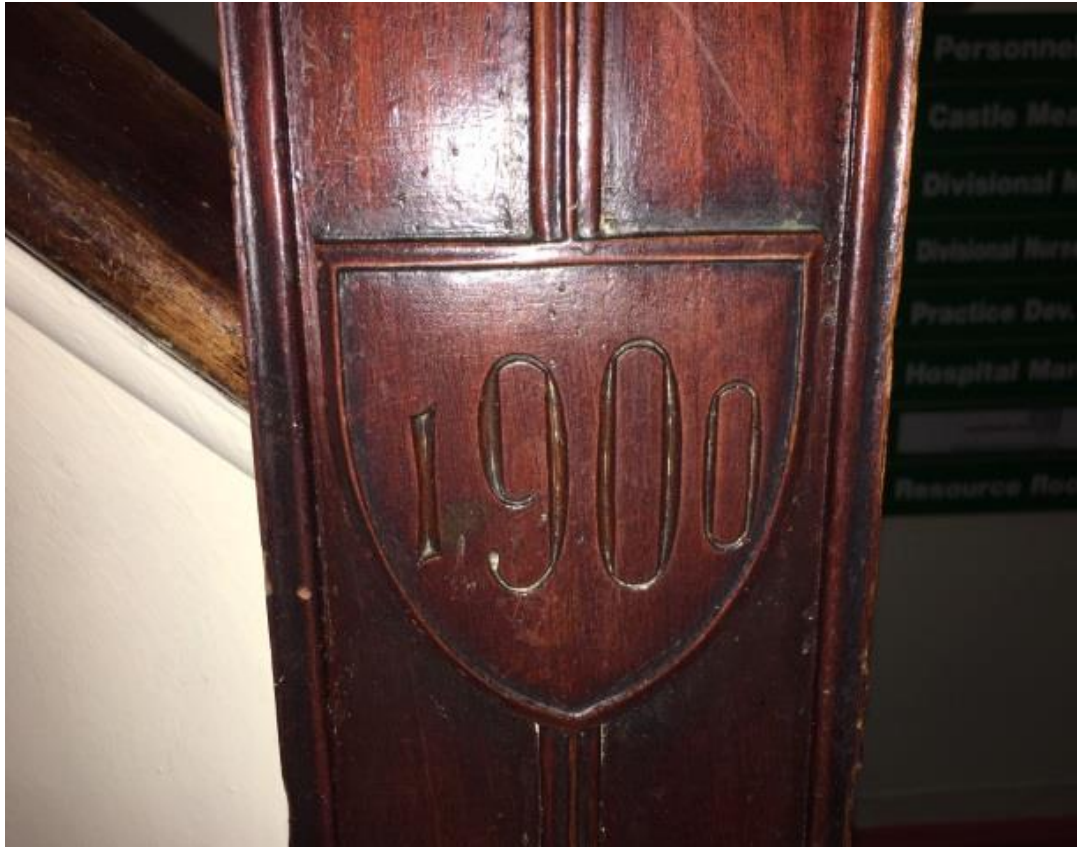
Photo 26 Date of original construction on stair post
