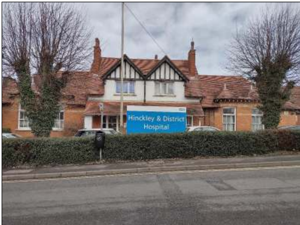
Photo 6 South-facing (principle) elevation of the Cottage Hospital
