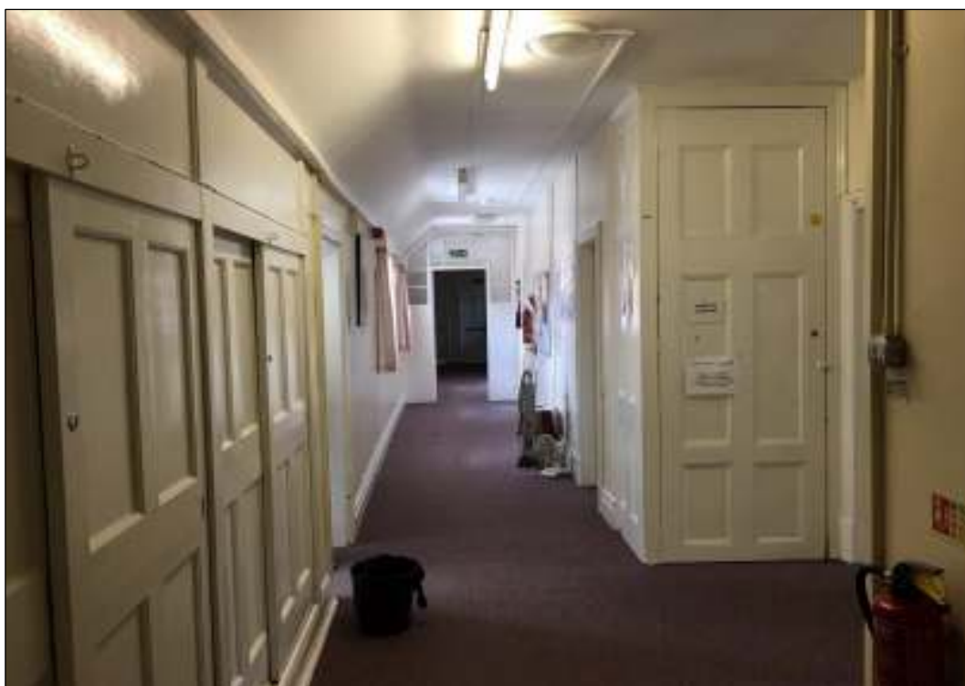
Photo 22 First floor central corridor
