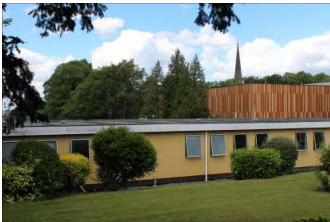
Photo 27 Temporary building to the west of the Cottage Hospital
