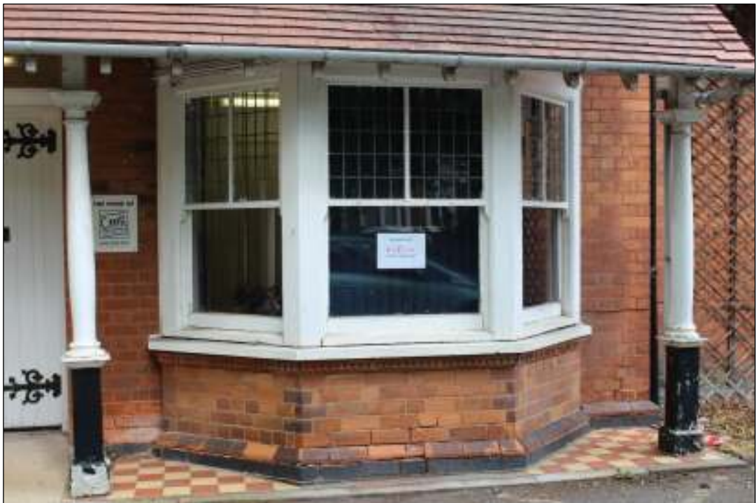
Photo 13 Bay window on principle entrance within the south-facing elevation (fronting onto Mount Road)
