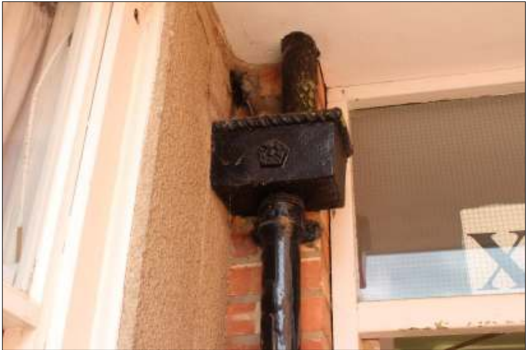
Photo 18 Cast iron rainwater goods with detail
