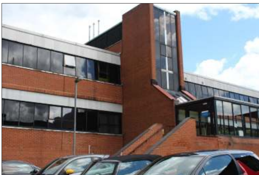
Photo 4 South-facing elevation of the Health Centre showing part of the glazed link to the Cottage Hospital
