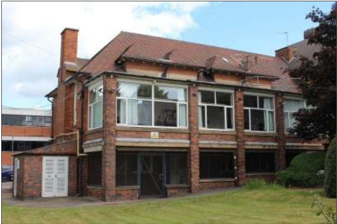
Photo 17 Current view of south-facing veranda windows on the north part of the west facing elevation, 1938 extension
