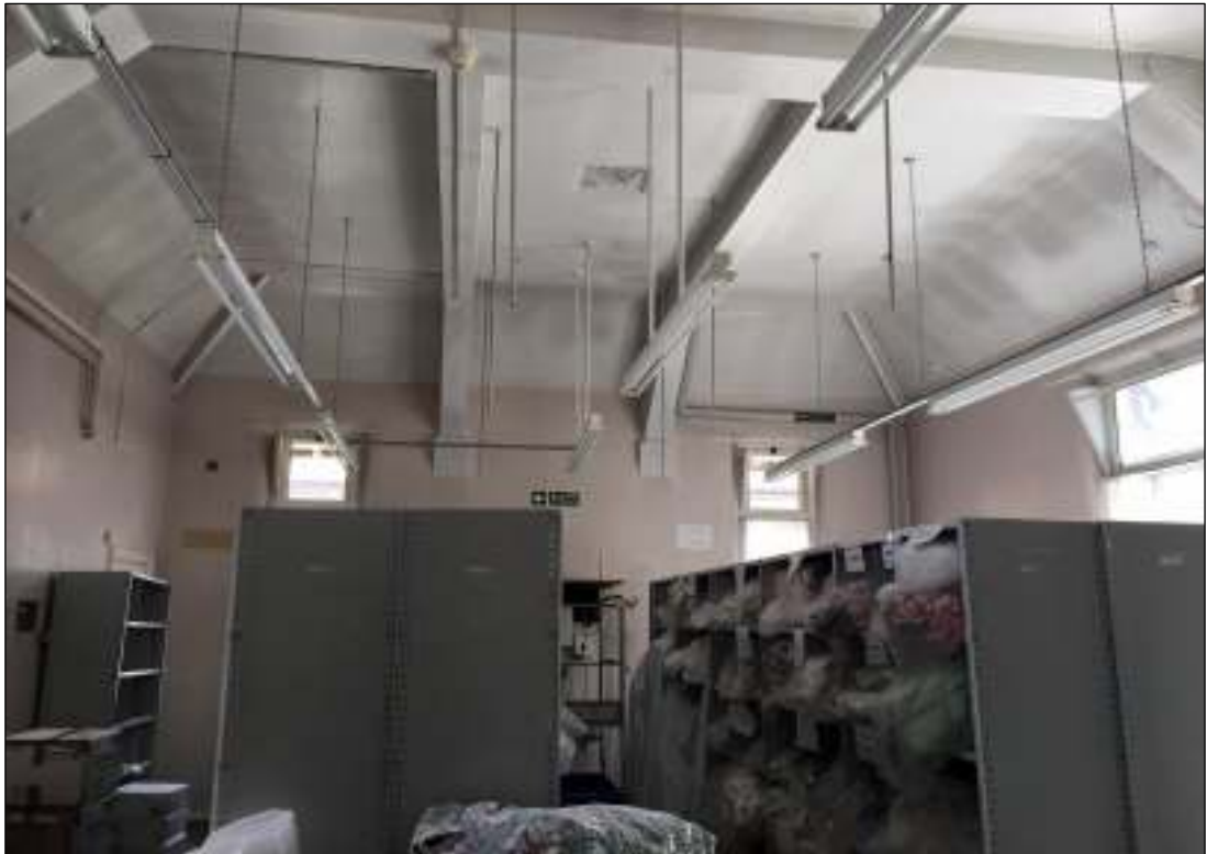
Photo 19 Original ward room to the right of the main entrance
