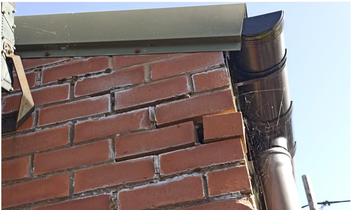
Plate 14: Image showing a gap in the brickwork along the north-west elevation of B3 , and the edge of some artificial lighting on the left-hand side.
