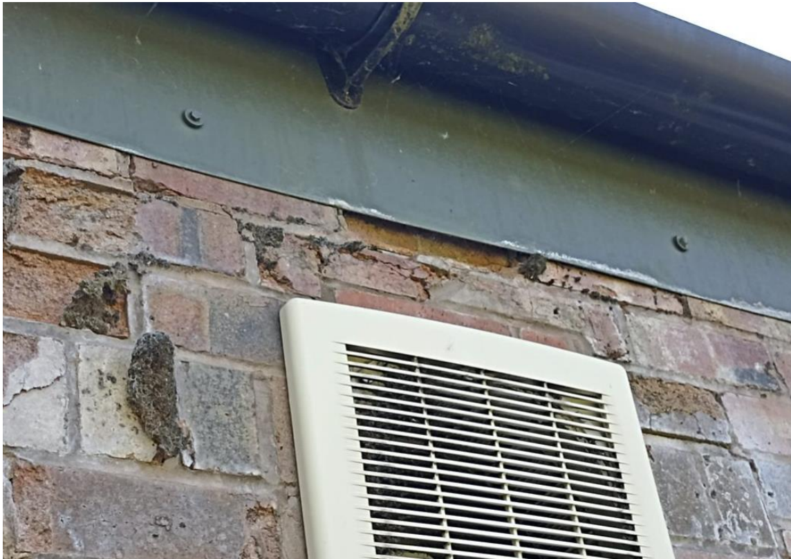
Plate 13: One of two gaps under the fasciae along the north-east elevation of B3 .
