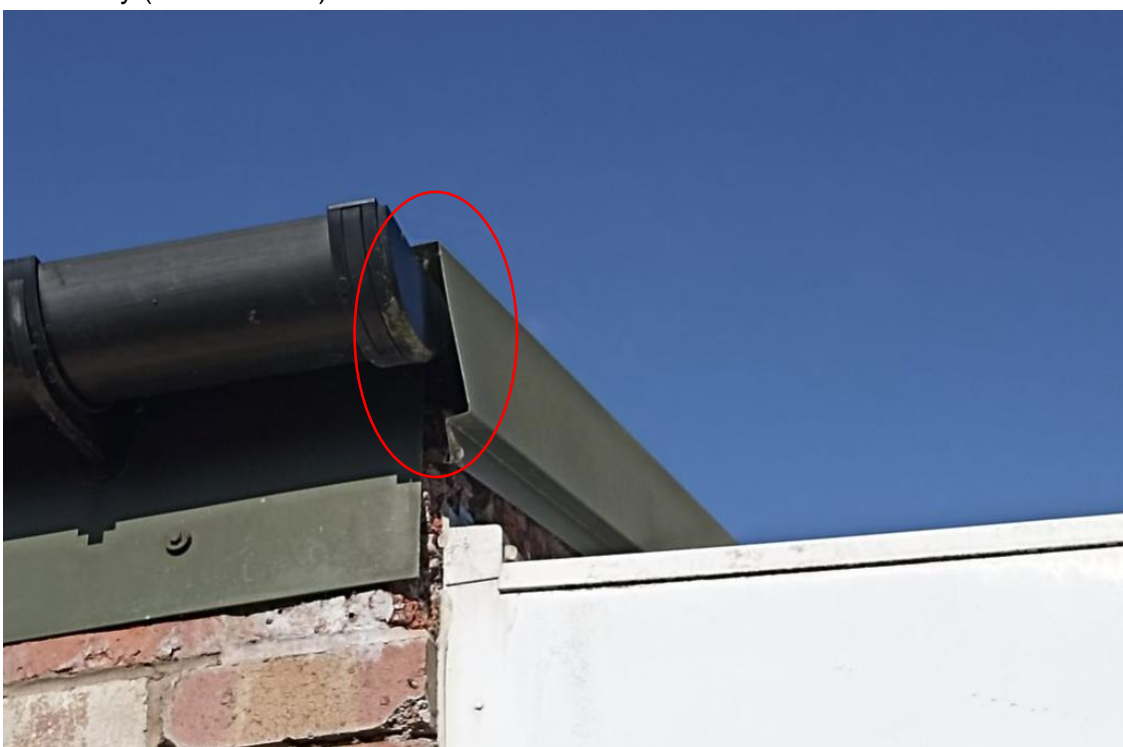
Plate 12: A gap under the bargeboard along the south-east elevation of B3 above the conservatory (circled in red).
