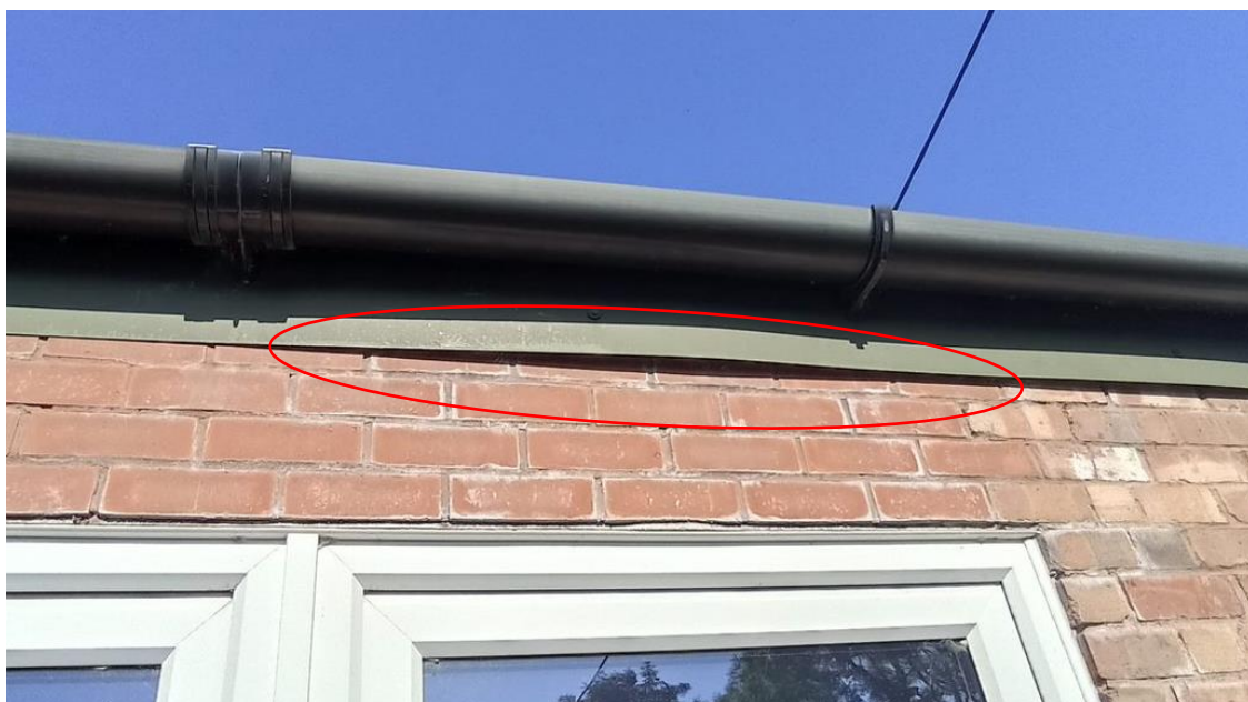
Plate 11: A gap under the fasciae along the south-west elevation of B3 (circled in red).
