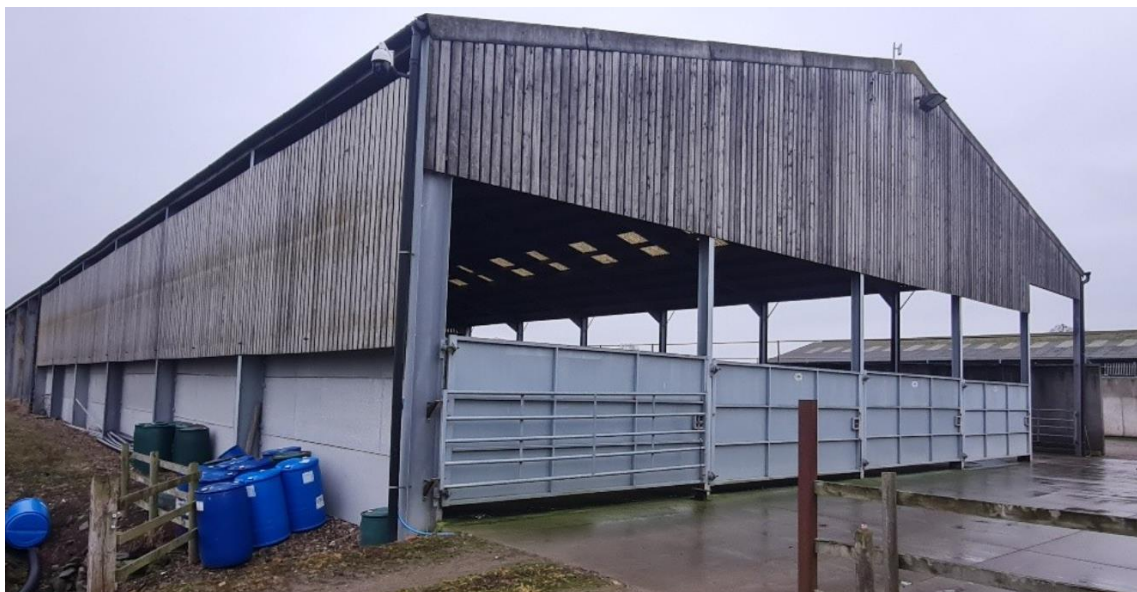
Figure 2 – north and east elevation
