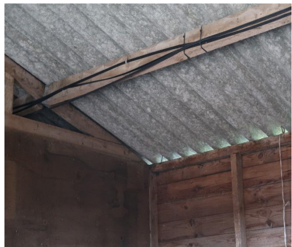
Internal view of stable block
