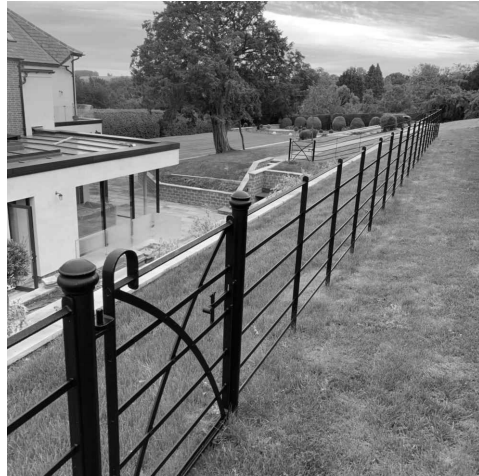
Metal Estate Fence/Gate
