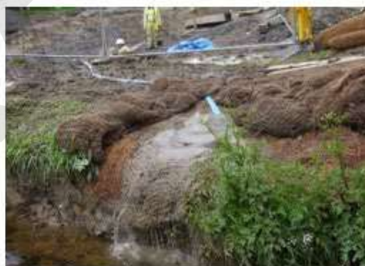
Deployed to treat muddy excavation water
