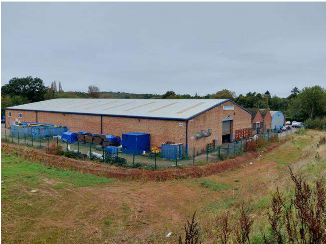
Photograph 4: View of site from south east corner
