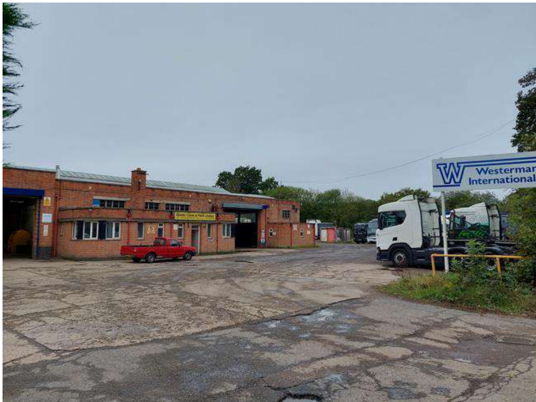
Photograph 2: View of Quinto Cranes Ltd unit from access
