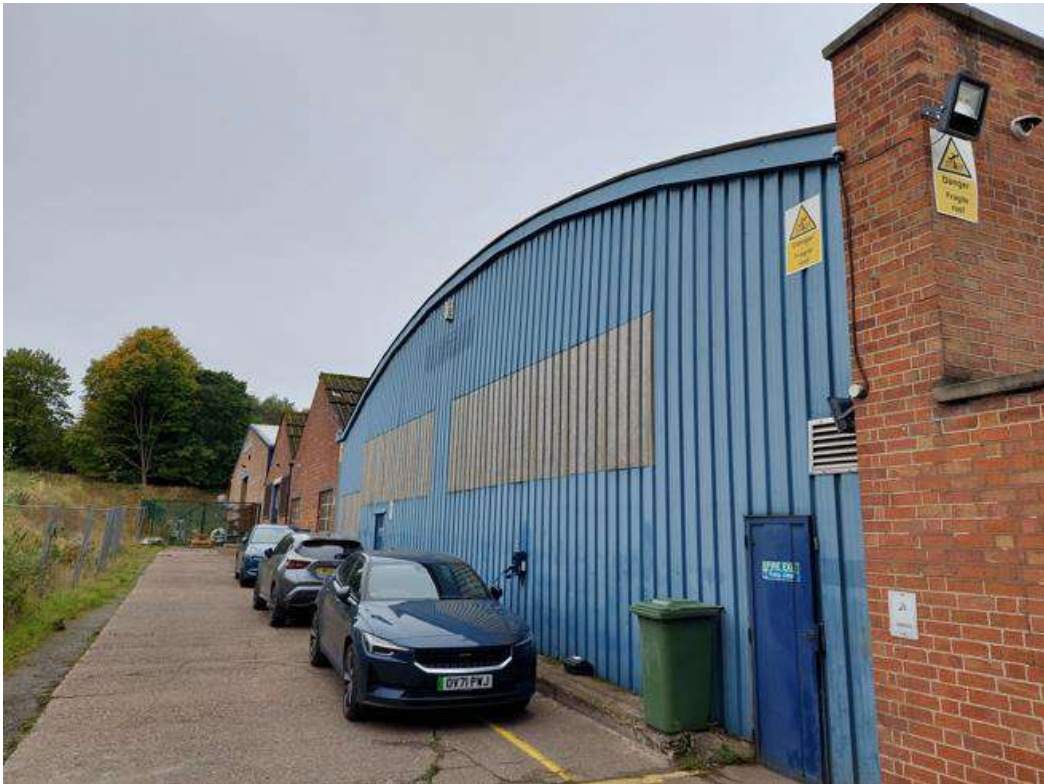
Photograph 3: View along eastern side of site, looking south
