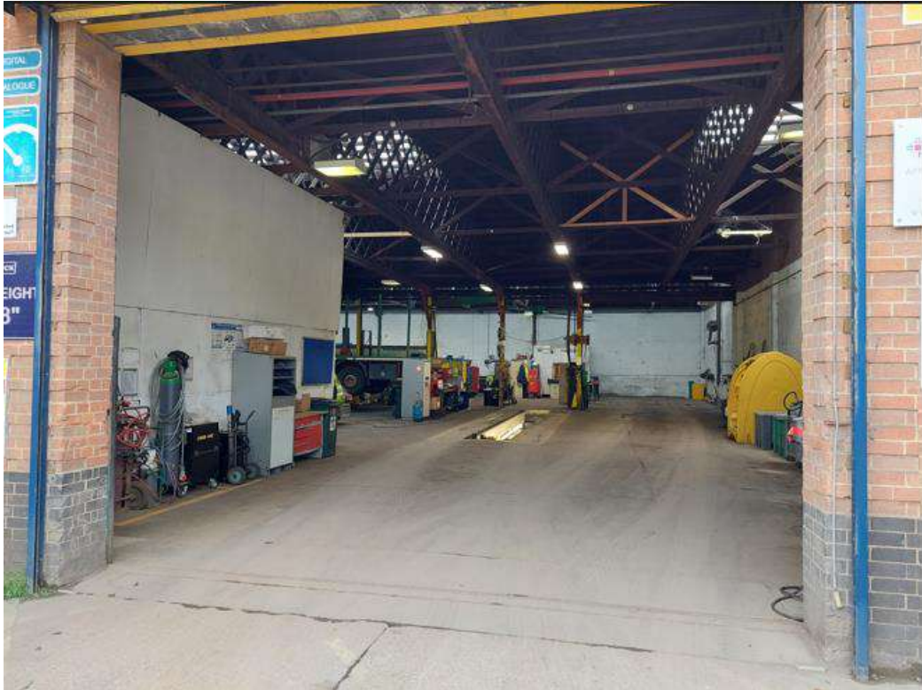
Photograph 9: View of internal area of Keltruck Ltd unit
