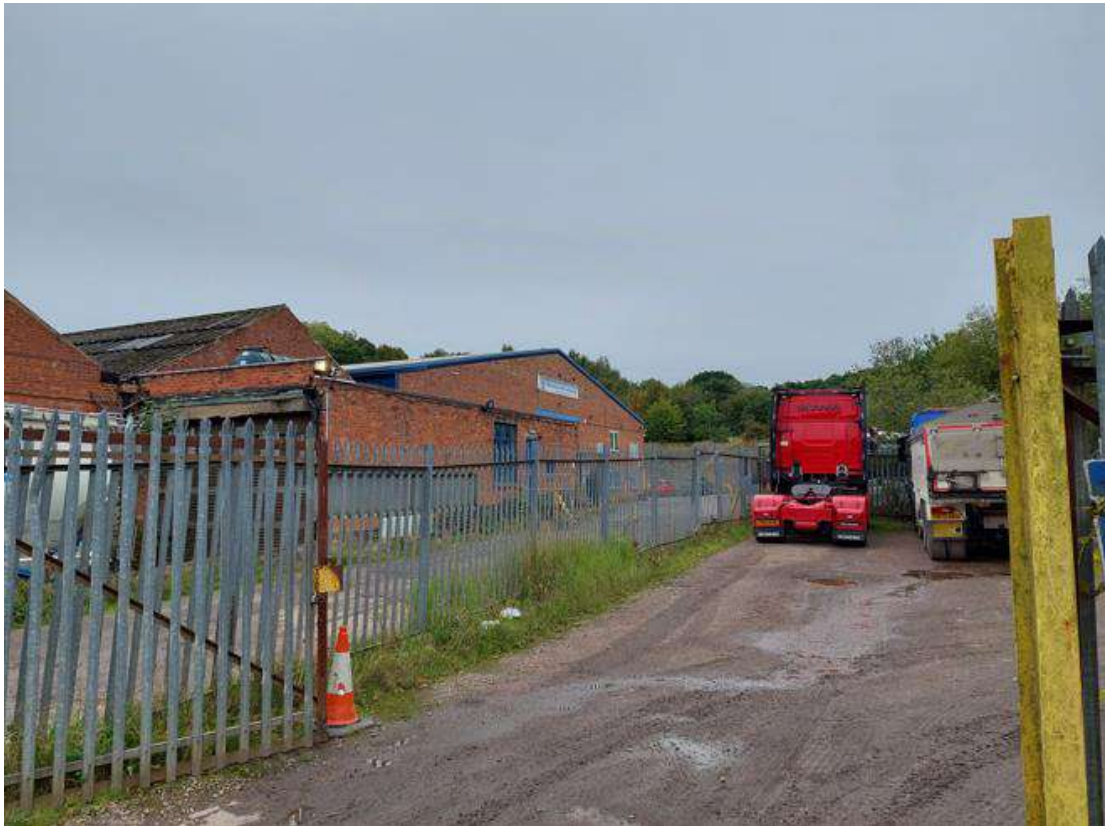
Photograph 14: Roof-located bulk fuel above ground storage tank and vehicle parking on western side of site
