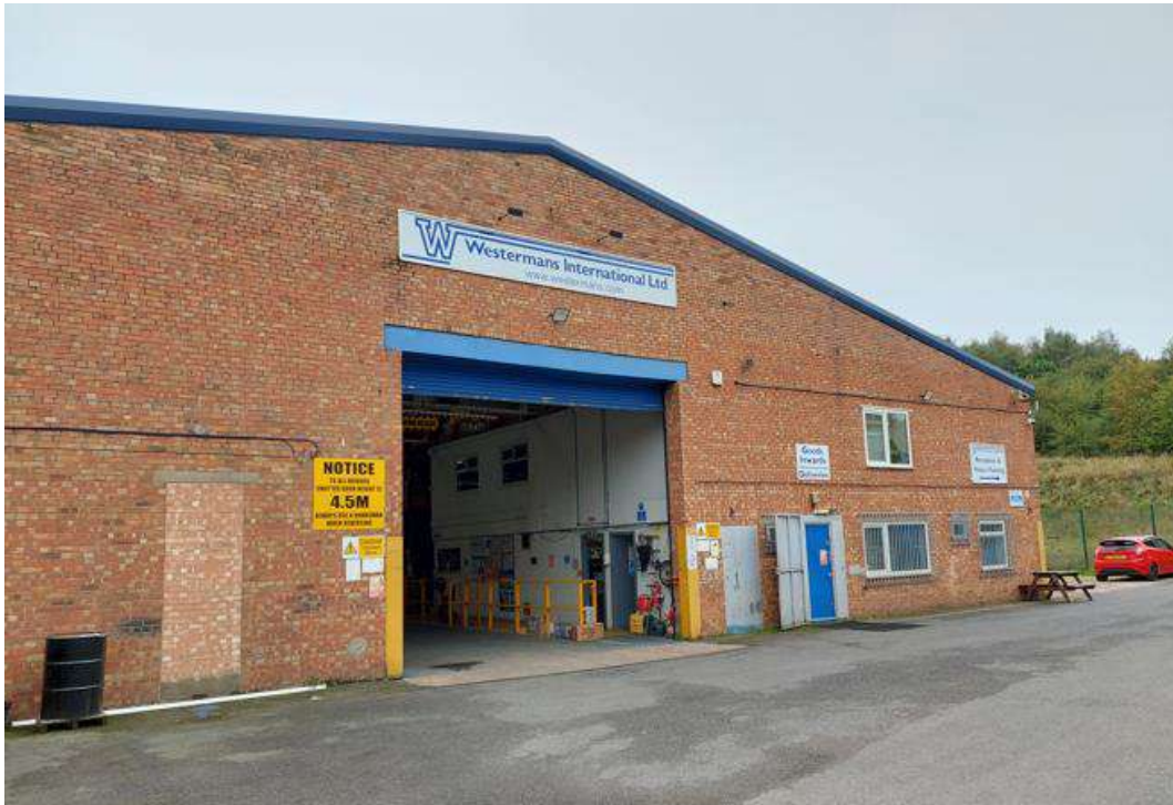
Photograph 11: Westermans International Ltd unit from western site boundary
